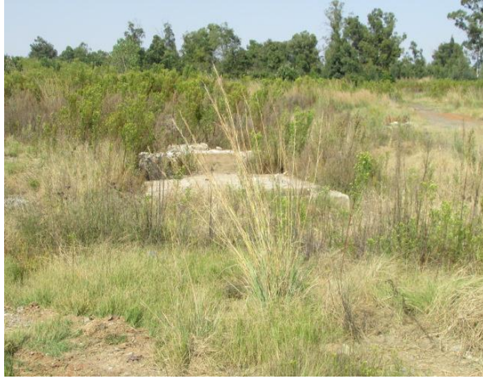
Fig.18: Foundations and ruins of old mining related structures close to Shaft 10.
