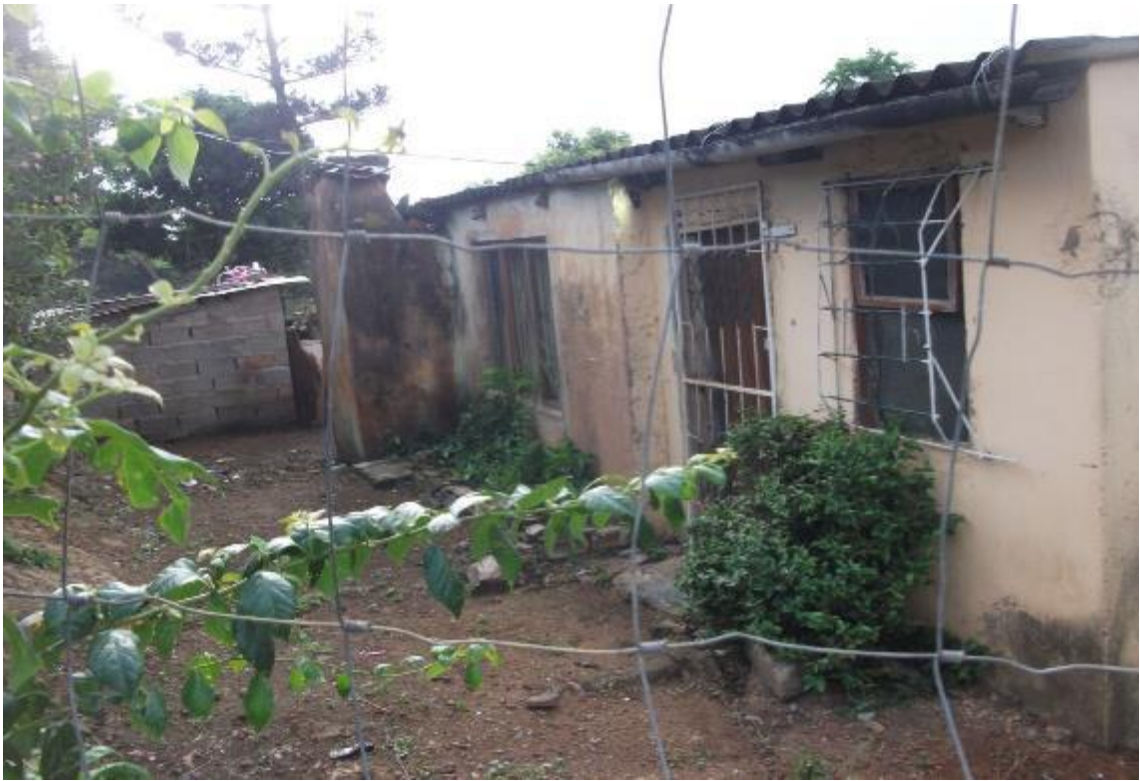
Figure 12: Structure potentially older than 60 years
