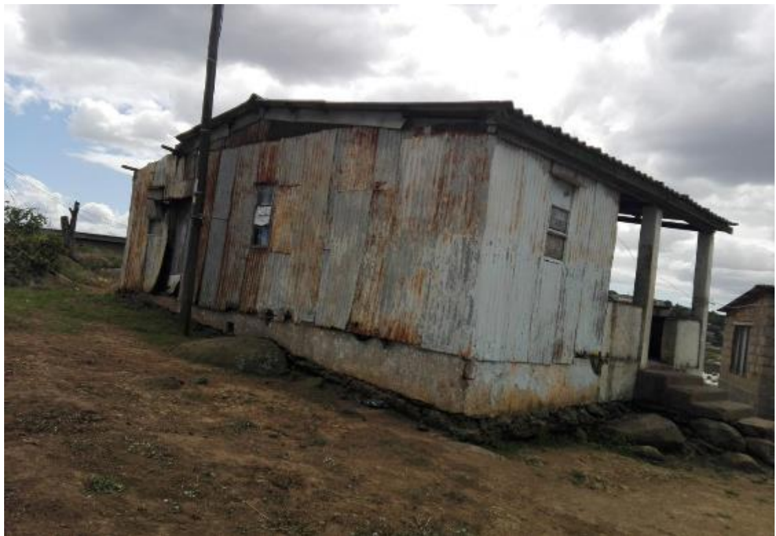
Figure 15: Corrugated iron house possibly >60 years
