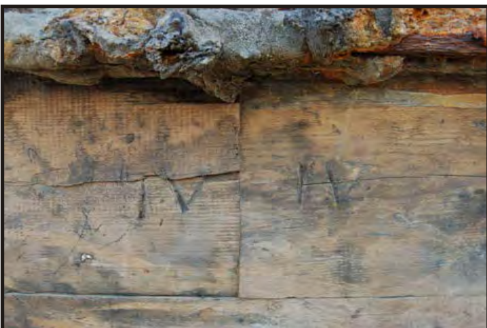
Figure 281: Ceiling marking - IV IV (Photo V. Maitland)
