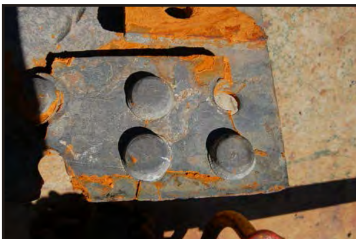
Figure 118: Top view of pan head rivets. (Photo V. Maitland)
