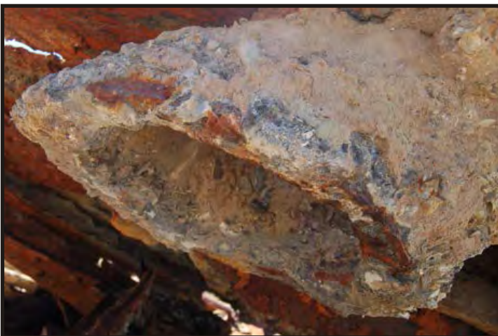
Figure 191: Side view of lower end of hawsepipe on the inner surface of the side plating. (Photo V. Maitland)
