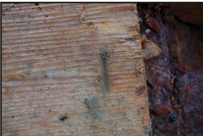
Figure 299: Ceiling marking - I (Photo V. Maitland)
