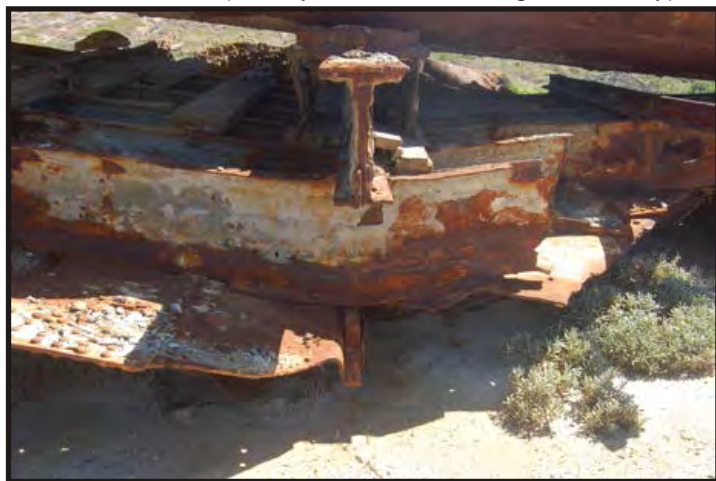
Figure 99: Floor showing bar keel, frames and keelson. (Photo V. Maitland)
