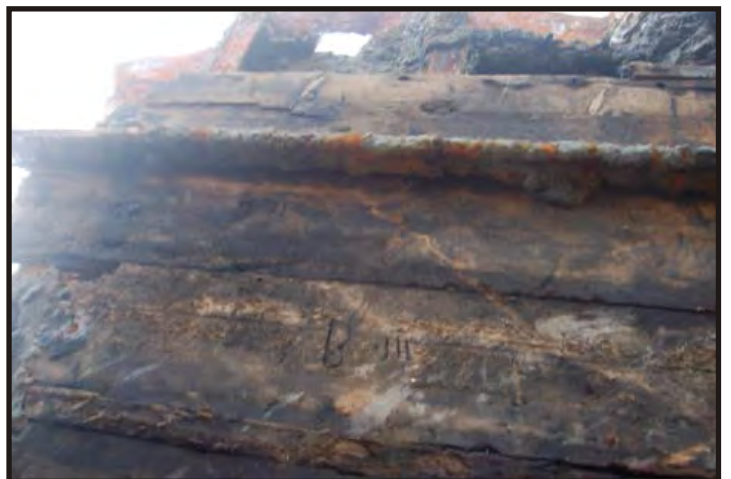
Figure 300: The ceiling in the hold shows the side stringers projecting above the ceiling. Thin filler planks are visible at the bottom of the photograph. (Photo V. Maitland)
