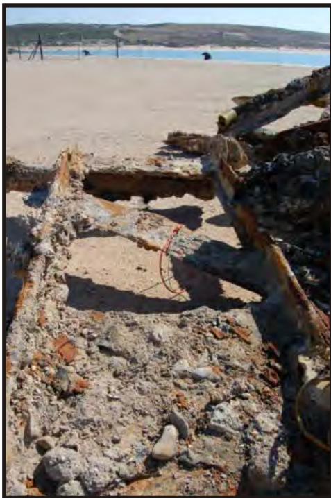
Figure 206: Part of a deck girder. (Photo V. Maitland)
