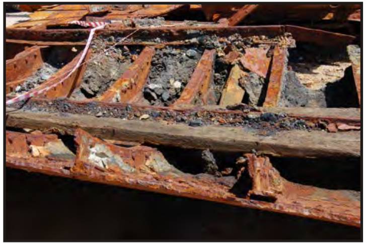
Figure 132: This view of the bilge shows the frames. The frames change from web frames on the floor to frame and reverse frames on the bilge and sides. (Photo V. Maitland)
