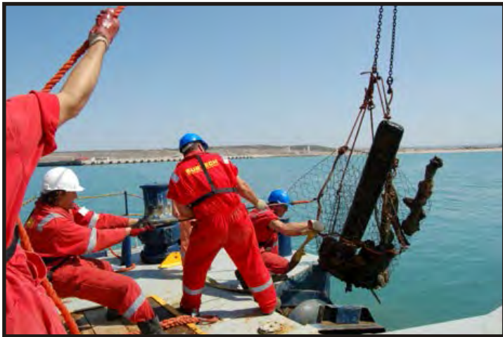
Figure 57: At first, wire gabions were used for lifting objects, however they were too weak and collapsed on retrieval. (Photo V. Maitland)
