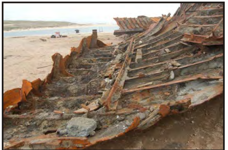
Figure 144: Side plating showing frames, side stringers and beam knees of the 'tween deck. (Photo V. Maitland)
