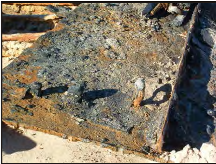
Figure 316: Close-up of rider plate and deck bolts. (Photo V. Maitland)
