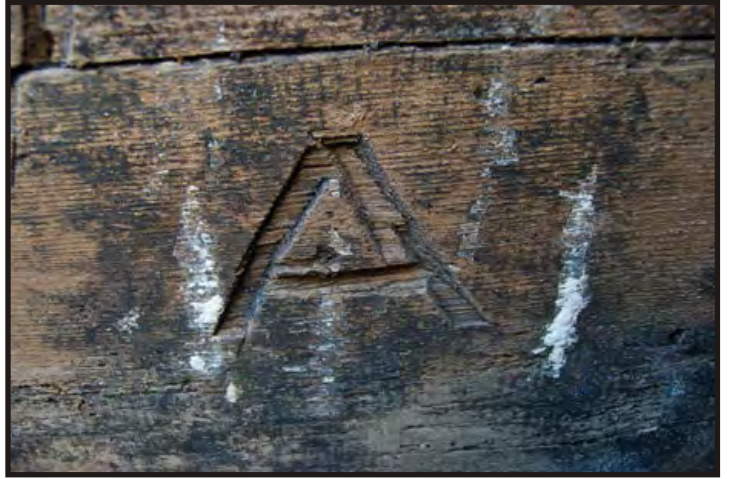
Figure 292: Ceiling marking - A II (Photo V. Maitland)
