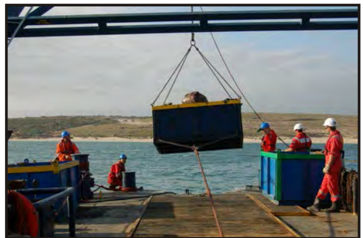
Figure 59 - 60: Metal bins were brought in to replace the gabions. These are very efficient as they lift large amounts and cause less damage to artefacts. (Photos V. Maitland)
