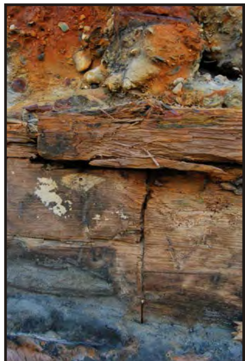
Figure 282: Ceiling marking - V V (Photo V. Maitland)
