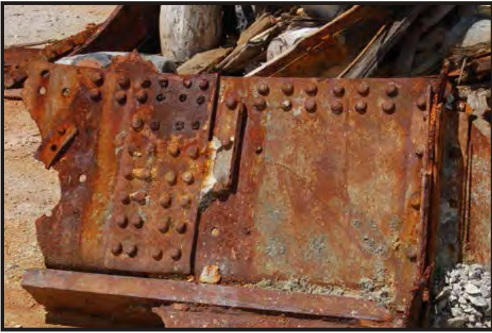
Figure 111: Section of the keel and garboard strake with a butt strap. (Photo V. Maitland)
