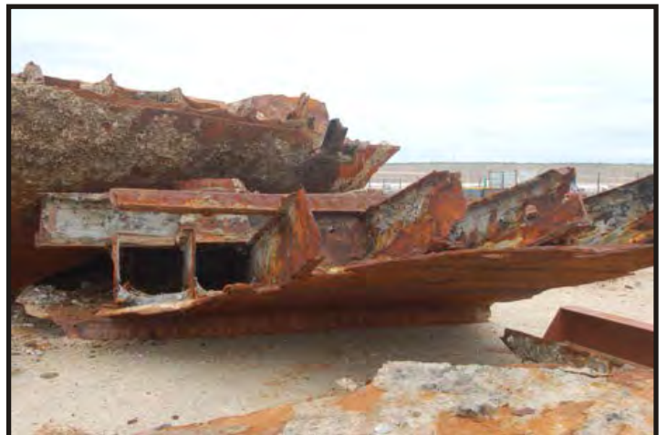
Figure 128: Side view of floor frames. (Photo V. Maitland)
