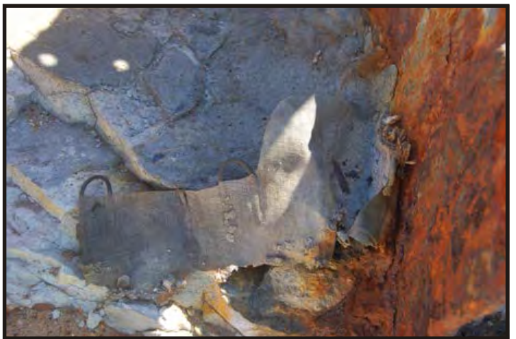
Figure 428: Underside of Figure 427. (Photo V. Maitland)
