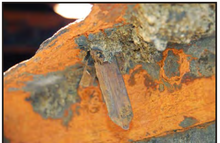
Figure 157: Bottom view of wooden dowel. (Photo V. Maitland)
