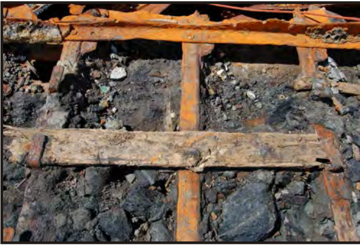
Figure 170: Side battens fixed in cleats. (Photo V. Maitland)
