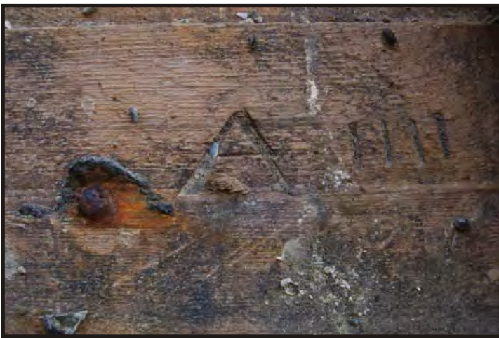
Figure 297: Ceiling marking - A III (Photo V. Maitland)
