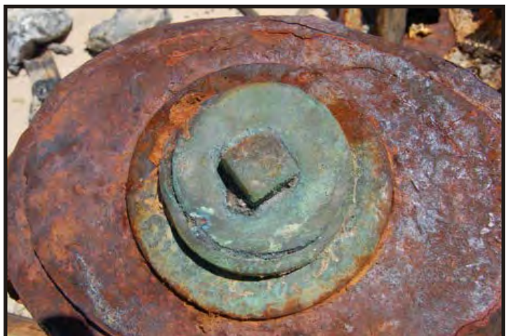
Figure 319: Close-up of the bollard top, with a square bolt and three brass 'washers'. (Photo V. Maitland)
