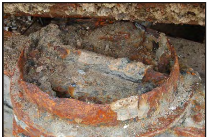
Figure 444: Close-up of the mast step. (Photo V. Maitland)
