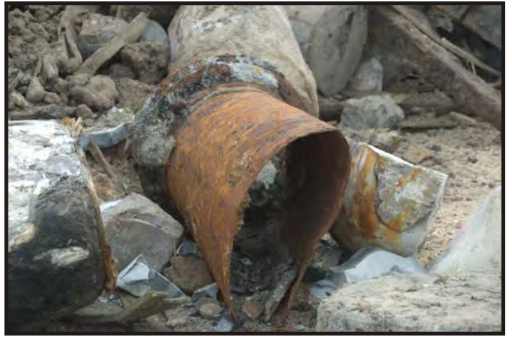
Figure 446: Mast heel. (Photo V. Maitland)
