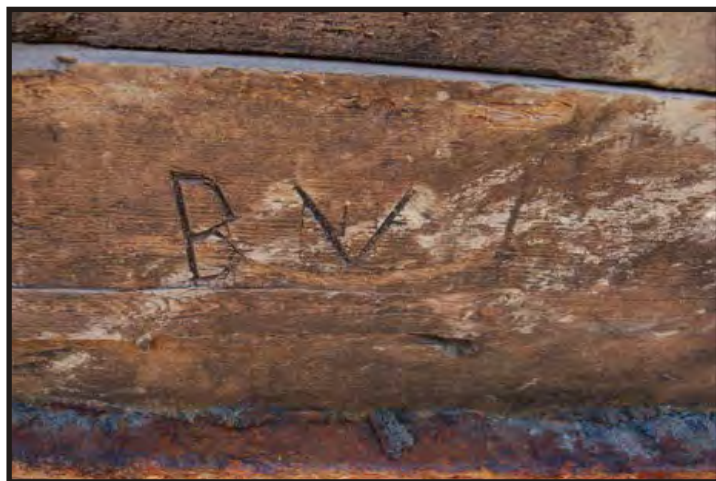
Figure 275: Ceiling marking - B V I (Photo V. Maitland)
