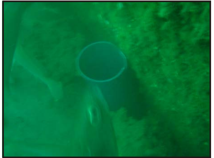
Figure 62: Conduit piping in the wreck for the charges. (Photo Subtech)
