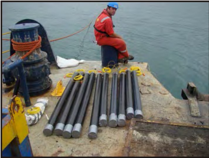
Figure 61: Explosive charges on the barge deck. Once all the loose material had been removed from the wreck site using dredging and manpower, Subtech used explosives to break up the conglomerated wreck. (Photo Subtech)
