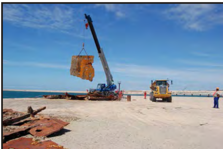
Figure 88 - 89: Large pieces of the hull being loaded onto a truck for transport to the dump site. (Photos V. Maitland)
