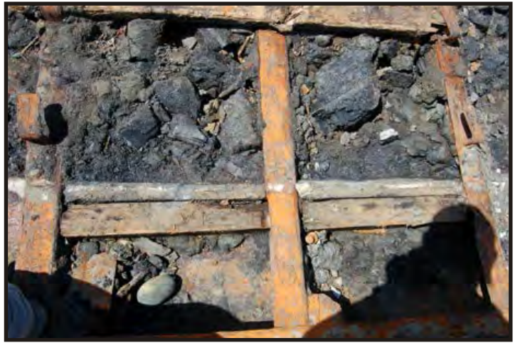
Figure 171: Additional dunnage was laid where water was likely to collect, including on stringers and stringer plates. Condensation would trickle down the plating and frames and lodge on the stringers (Brown 1931:391). Marked from left to right with Roman numerals, VI and VII. (Photo V. Maitland)
