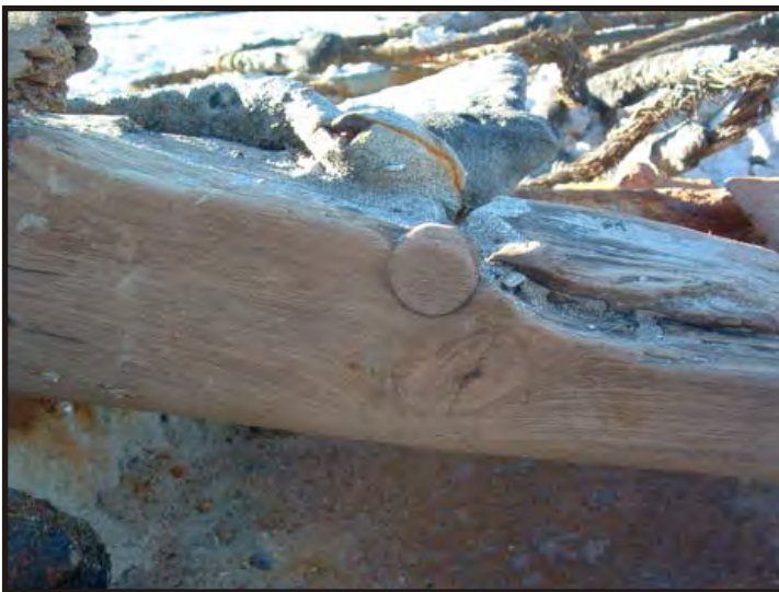
Figure 226: Top of gunwale and dowel covering the bolt. (Photo V. Maitland)
