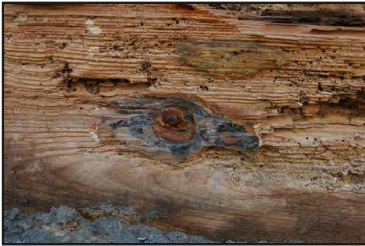
Figure 302: The ceiling was attached to frames with iron bolts. (Photo V. Maitland)
