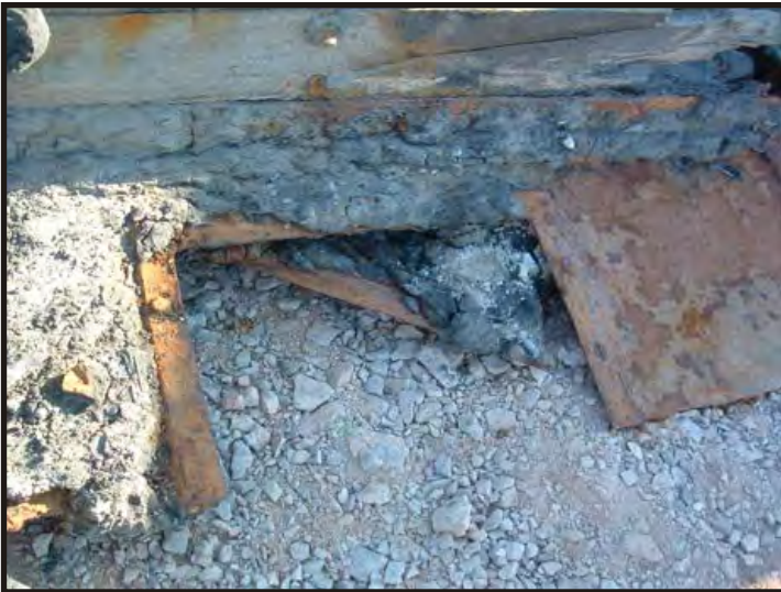
Figure 235: Scupper on the bulwark under the channel. (Photo V. Maitland)
