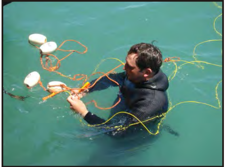
Figure 64: Organising the shock tubes to the charges. (Photo Subtech)
