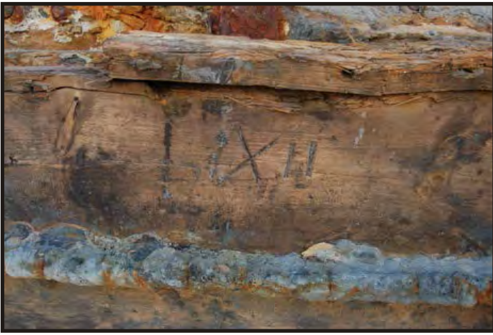
Figure 277: Ceiling marking - XII (Photo V. Maitland)
