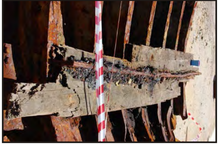
Figure 153: Ceiling next to the side keelson. (Photo V. Maitland)
