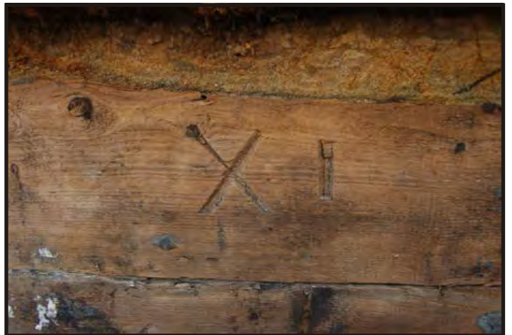
Figure 288: Ceiling marking - XI (Photo V. Maitland)
