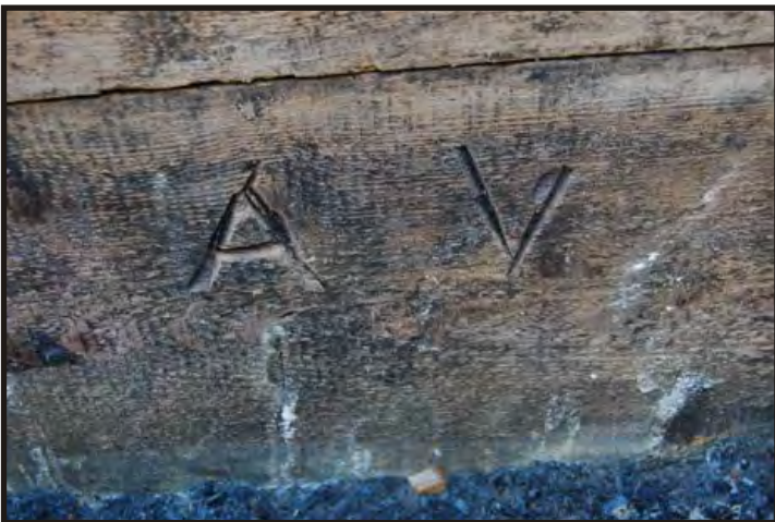
Figure 287: Ceiling marking - AV (Photo V. Maitland)
