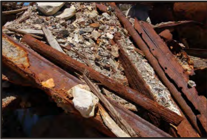
Figure 182: Pillars at the dump site. (Photo V. Maitland)
