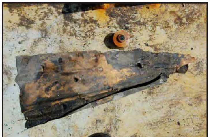
Figure 417: Copper sheeting. This was used to cover repairs to the wood. (Photo V. Maitland)
