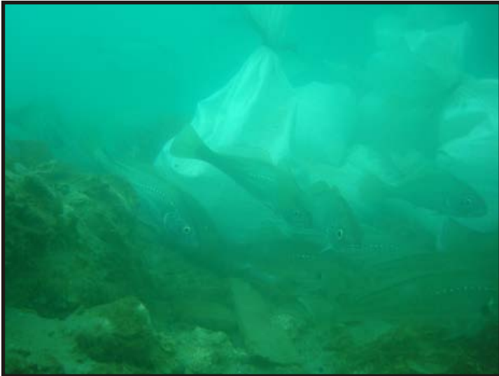
Figure 63: Sandbags packed onto the wreck to contain and control the direction of the blast. (Photo Subtech)
