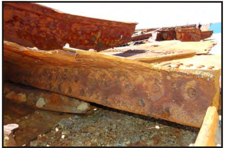
Figure 123: Zig-zag riveting on the keel. (Photo V. Maitland)
