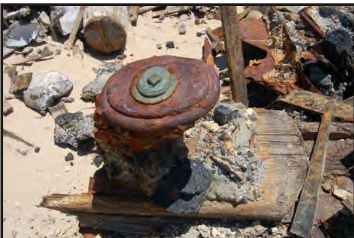
Figure 318: Top view of the bollard. The shaped bollard plank attached to the deck is visible. (Photo V. Maitland)
