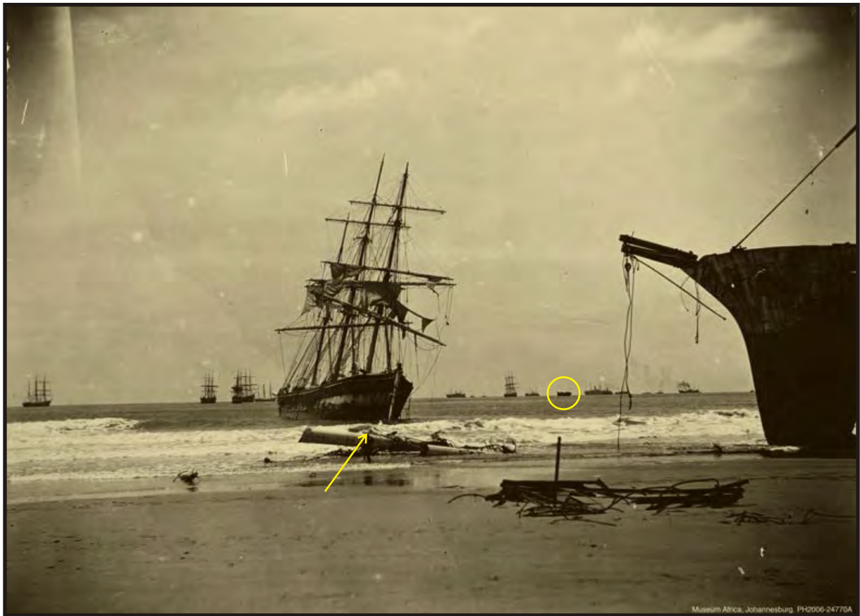
Figure 32: The bow of the vessel in the foreground is the Emmanuel . In this photograph the County of Pembroke 's bowsprit has fallen off, the side of the figurehead is visible. The sails are slightly unfurled as per the eyewitness accounts and the masts and spars are white as per Bisset's description. The vessel circled in the background is probably the hull of the dismasted Lütto .
