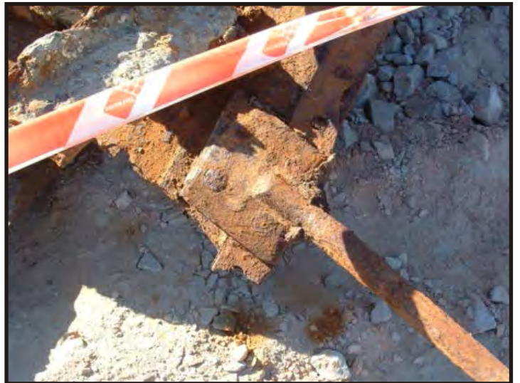
Figure 238: Close-up of chain plate where it's riveted to the bulwark. (Photo V. Maitland)
