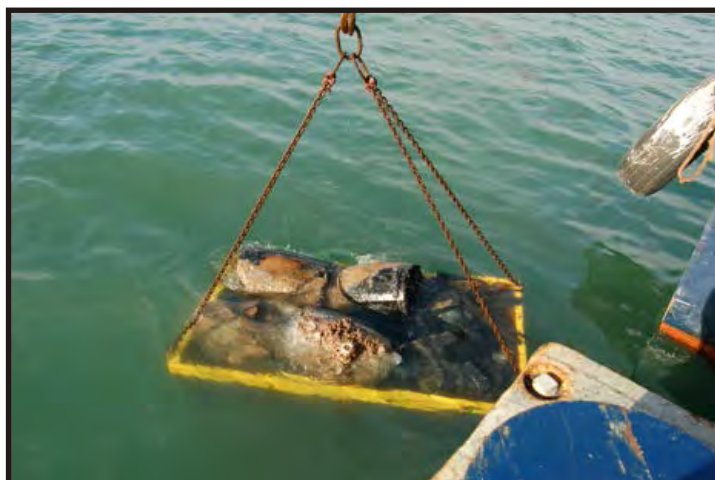
Figure 59 - 60: Metal bins were brought in to replace the gabions. These are very efficient as they lift large amounts and cause less damage to artefacts. (Photos V. Maitland)
