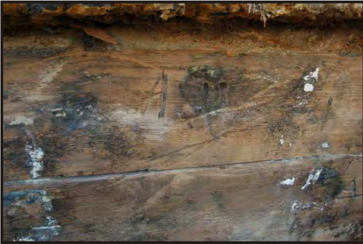
Figure 285: Ceiling marking - AII (Photo V. Maitland)
