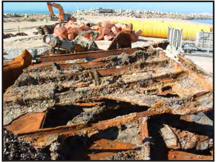
Figure 204 - 205: Two different views of the underneath of part of a deck girder. (Photo V. Maitland)
