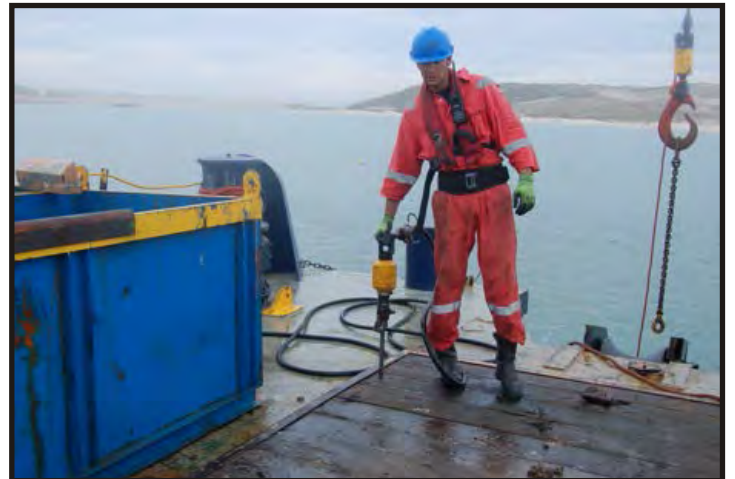
Figure 58: A hydraulic underwater jack hammer is used to break up large sections of conglomerate. (Photo V. Maitland)
