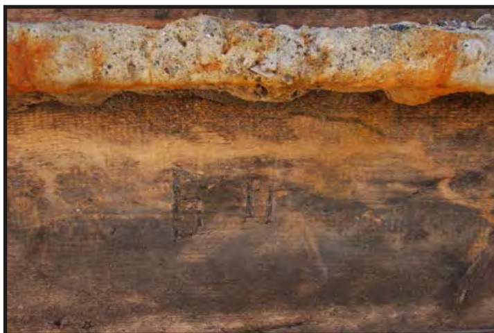
Figure 272: Ceiling marking - B II (Photo V. Maitland)
