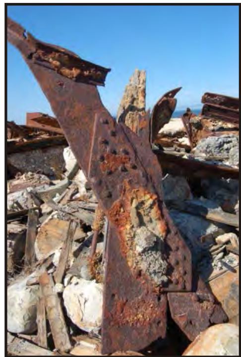
Figure 207: Close-up of the diagonal tie plates. (Photo V. Maitland)
