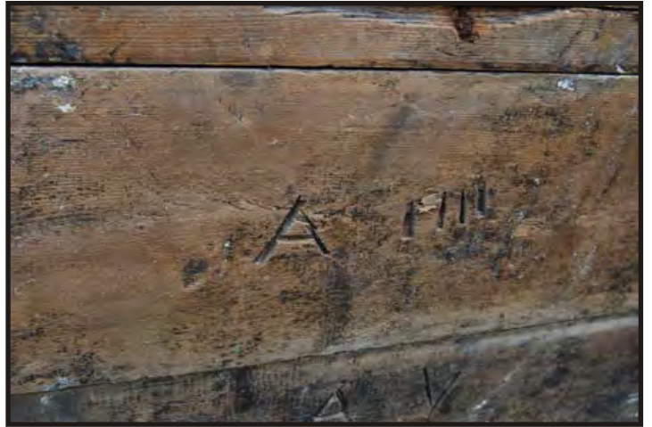
Figure 286: Ceiling marking - AIII (Photo V. Maitland)
