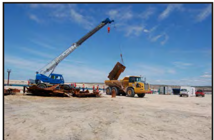
Figure 88 - 89: Large pieces of the hull being loaded onto a truck for transport to the dump site. (Photos V. Maitland)
