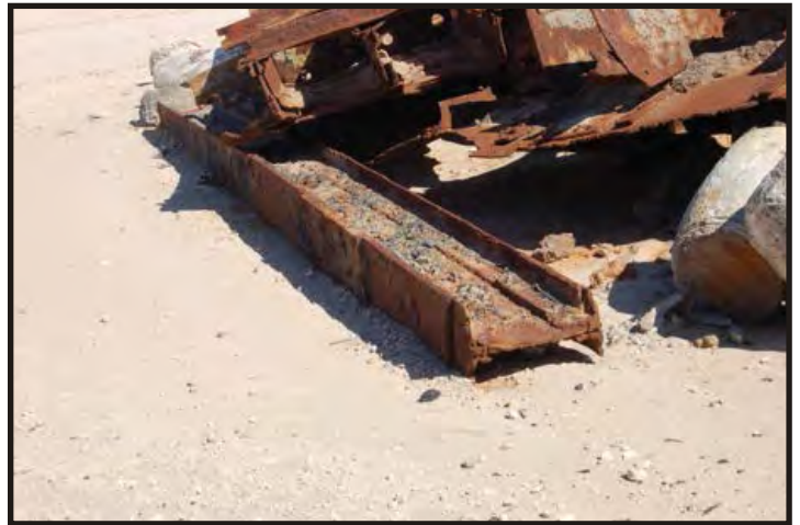
Figure 149: Built H-beam. These were used where strong support was required. (Photo V. Maitland)
