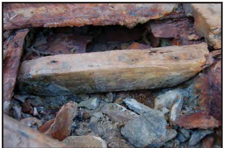
Figure 305: Intercostal wooden block. (Photo V. Maitland)
