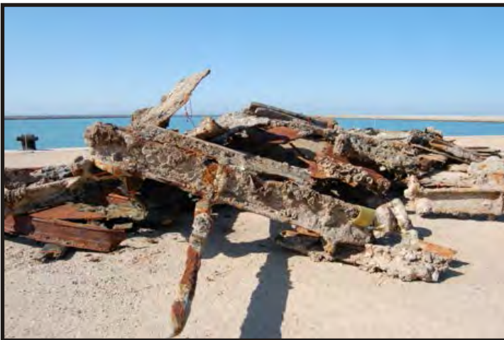
Figure 178: Pillar attached to the deck beam. (Photo V. Maitland)
