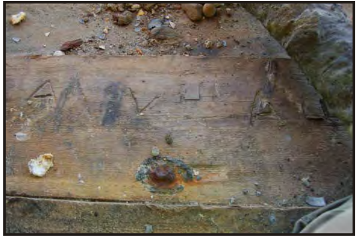
Figure 296: Ceiling marking - A V III A III (Photo V. Maitland)
