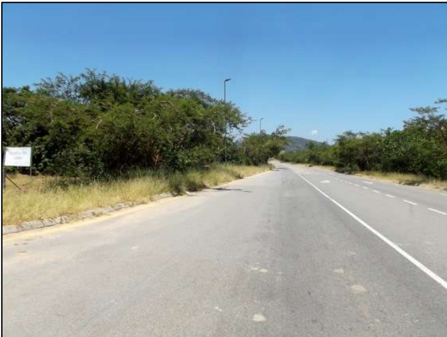
Fig. 8. Site SO 1. Photo taken in a south western direction.
