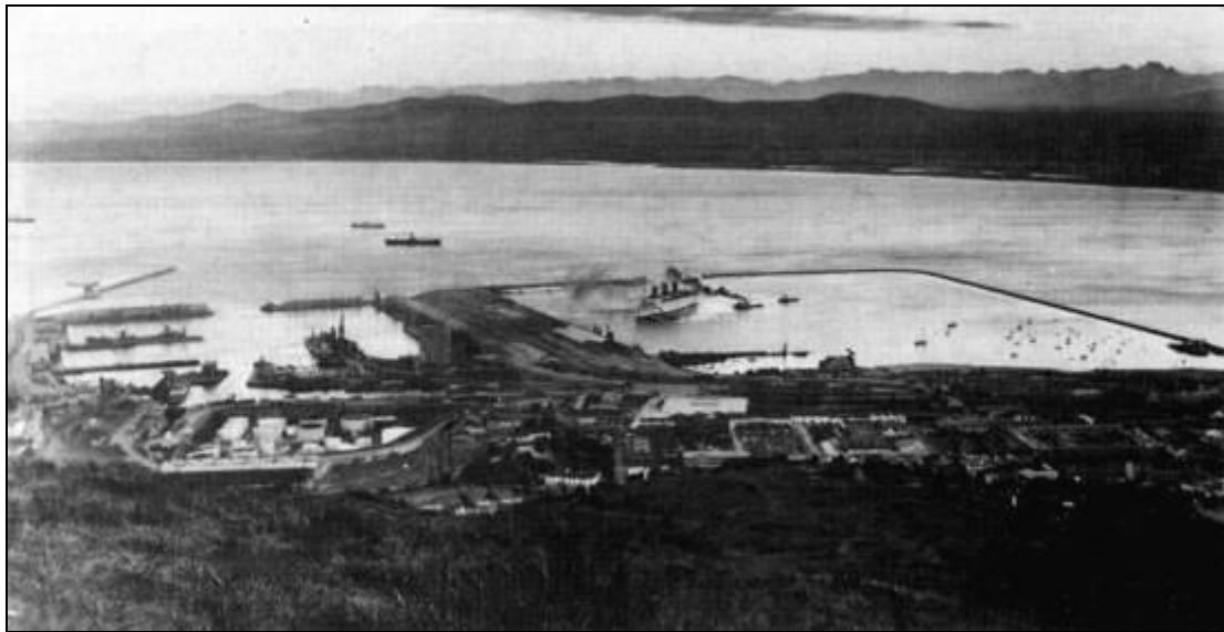
Figure 11: The new southern basin in 1934 with the random block mole at right 21
