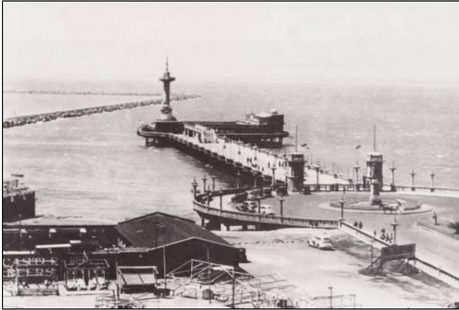
Figure 10: The 1913 municipal pier at the foot of Adderley Street. The random block mole can be seen at left 18
