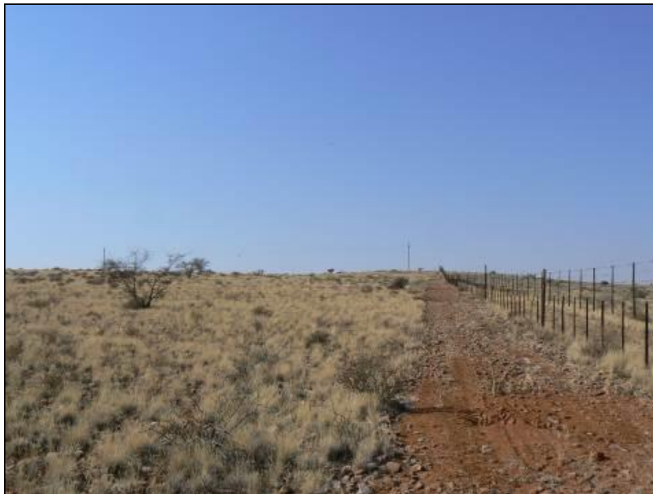
FIGURE 5: General view along the western boundary fence looking south
