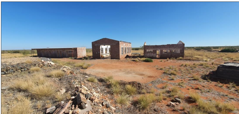
Figure 9: General view of the existing infrastructure in the survey footprint (northern section)
