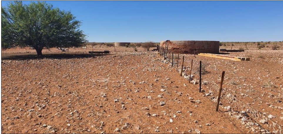
Figure 16: General view of existing infrastructure western section of the survey footprint
