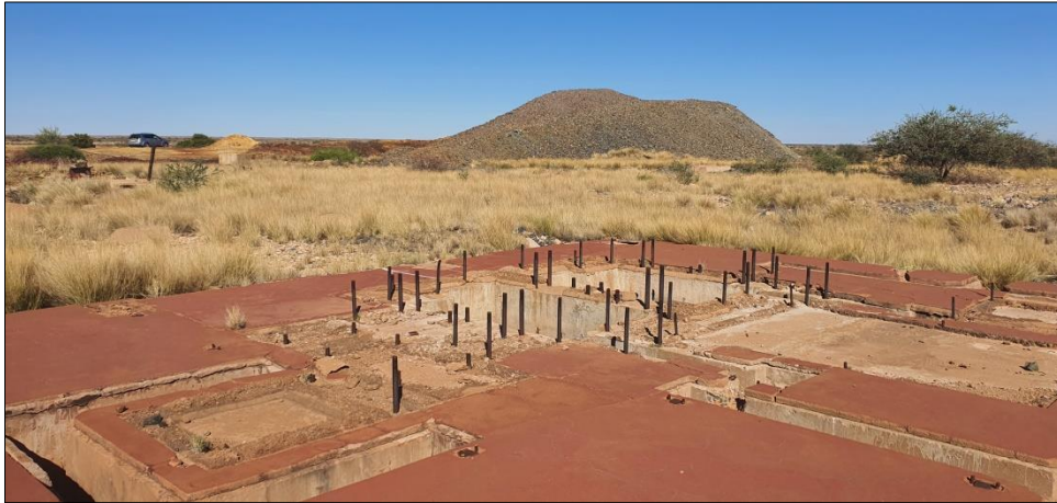
Figure 10: General view of the existing infrastructure in the survey footprint (northern section)
