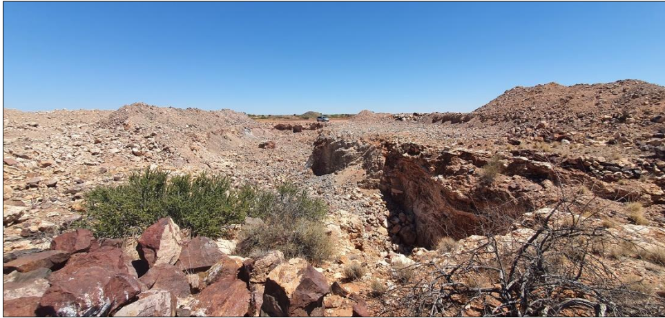
Figure 13: General view of the previous mining activities in the southern section of the survey footprint
