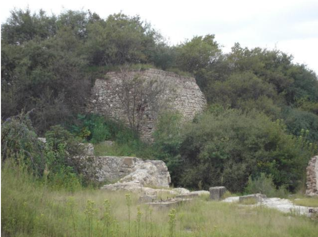
No. 2 Remains of the lime works
