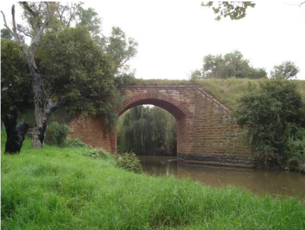
No. 12 The sandstone Bridge over the Kaalspruit
