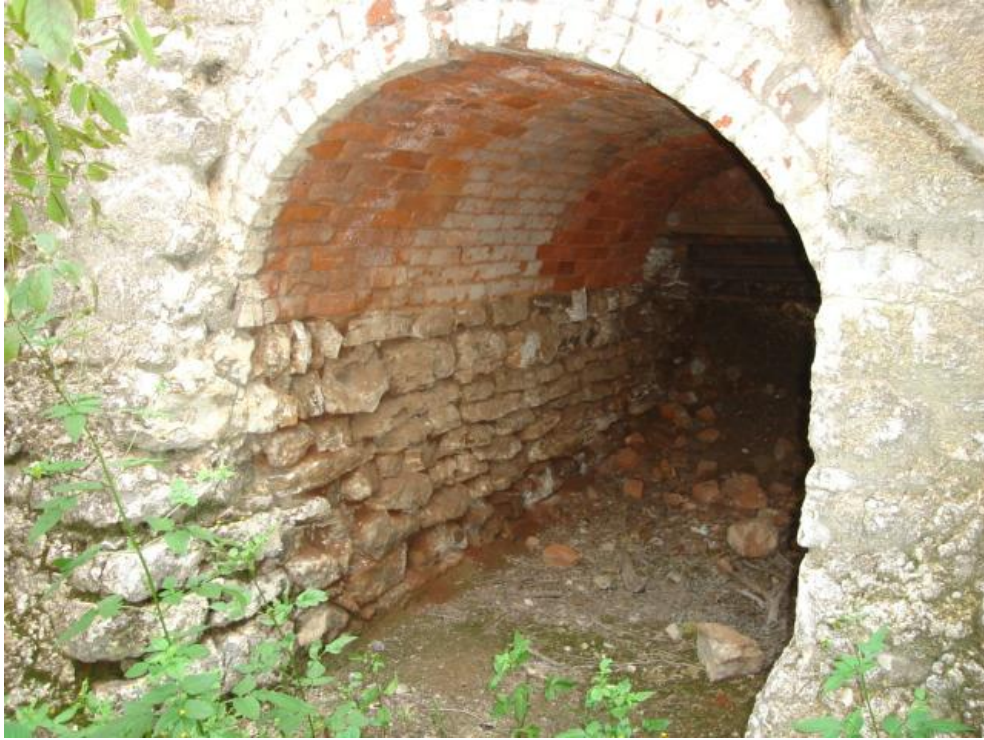
No. 3 Detail of the lime kilns
