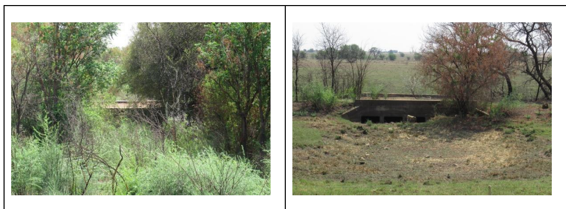
Figure 11. Views of the two old bridges
