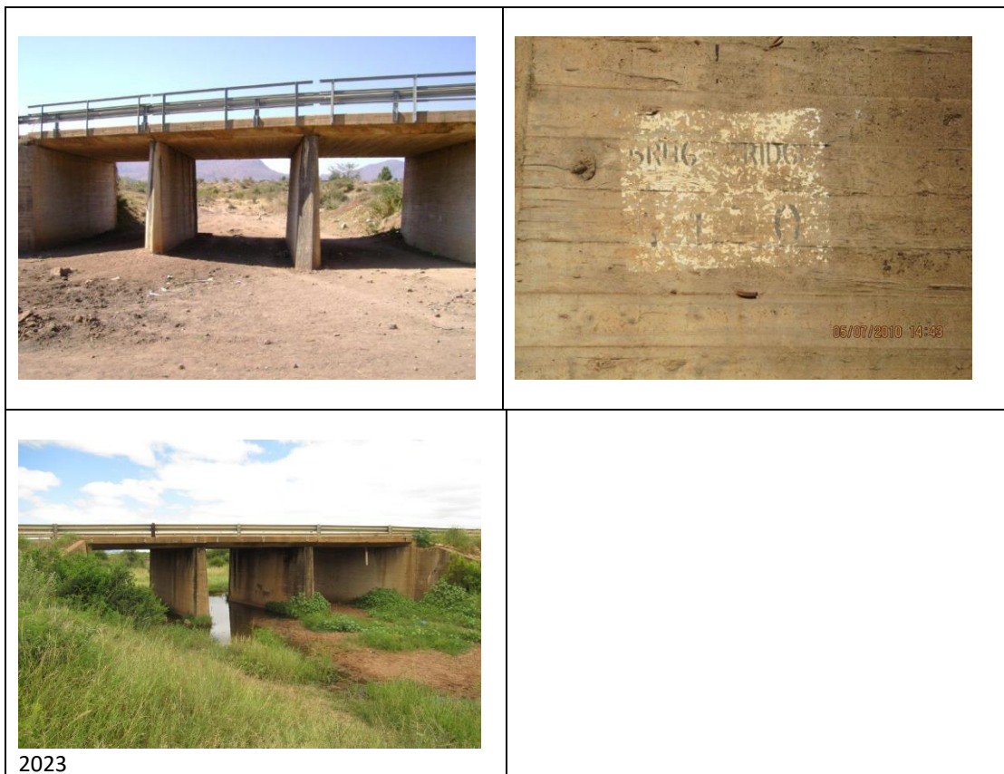
Fig. 13. Side-view of the bridge and its identification number.
