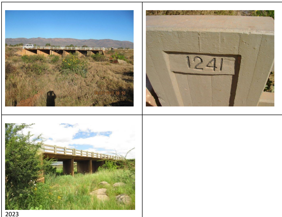
Fig. 10. Side-view of the bridge and its identification number.
