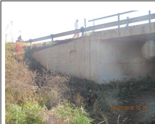
Abutment wall, north-eastern side
