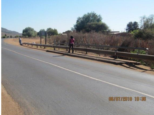
Bridge deck seen from the top
