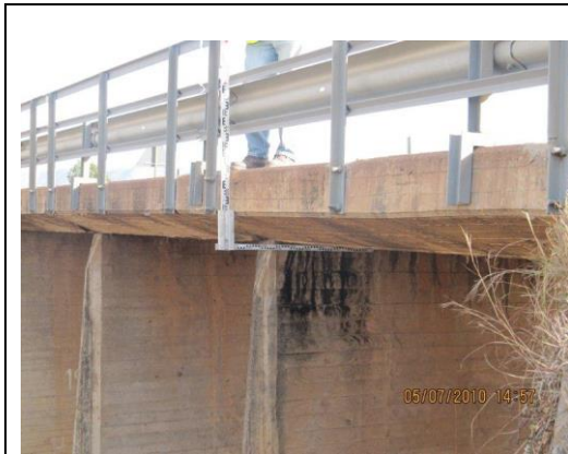
Railing on eastern side of bridge
