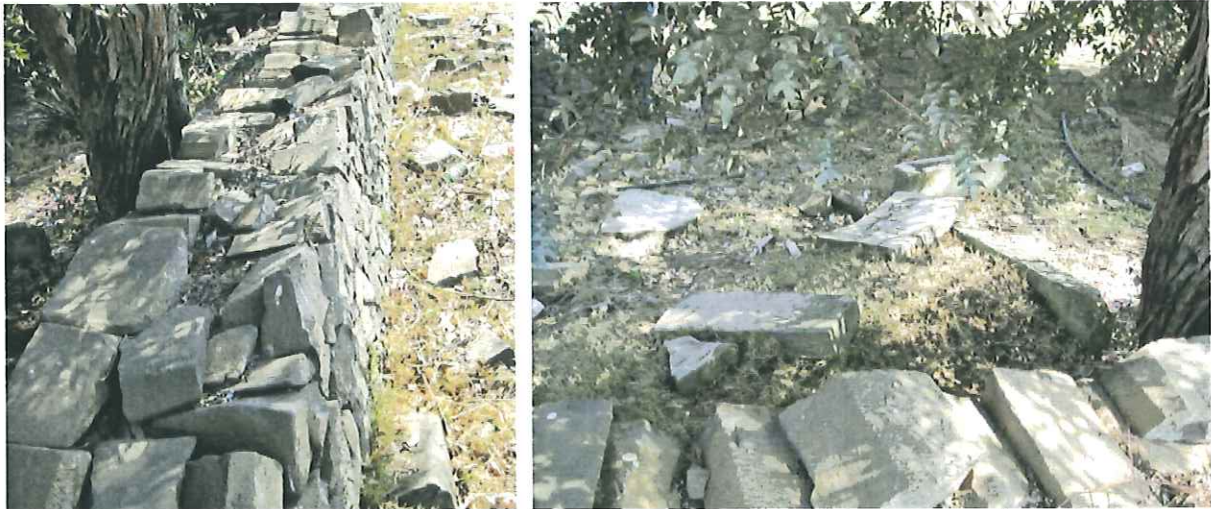
Figure 7. The Roets family cemetery. Note the masonry in the wall and the desecrated graves.
