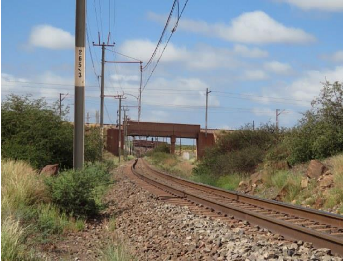
Figure 3: Part of the existing railway infrastructure in the vicinity.
