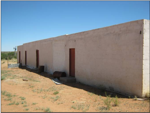
Figure 21: View of the front of the farm building.
