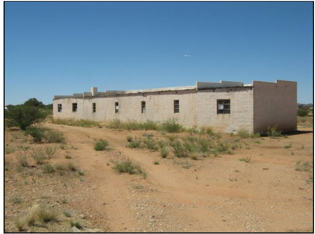
Figure 22: View of the rear of the farm building.
