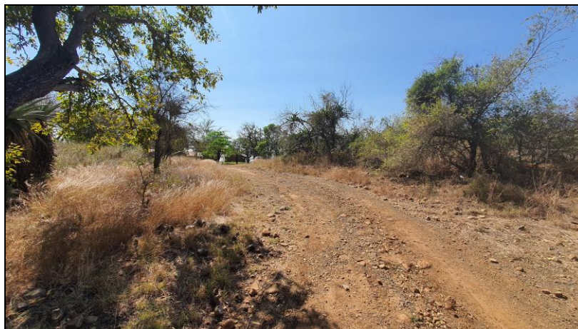
Figure 7: General view of the existing infrastructure in the southern section of the survey footprint
