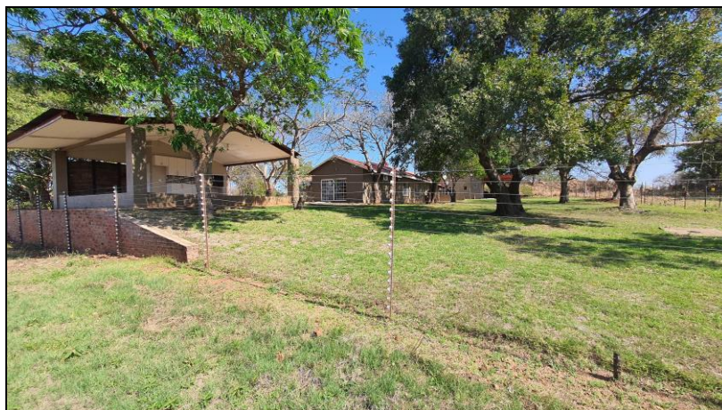
Figure 8: General view of the existing infrastructure in the southern section of the survey footprint
