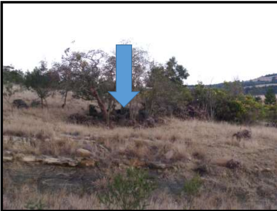
Figure 6. Local residents thought that potential graves occur in the bushes (indicated by the blue arrow). However, investigations by the consultant indicated that the actual graves are situated more than 50m from the D 1269 and these are not threatened by the proposed development
