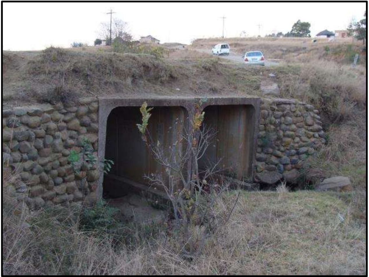
Figure 11: Concrete box culverts at water crossing 3
