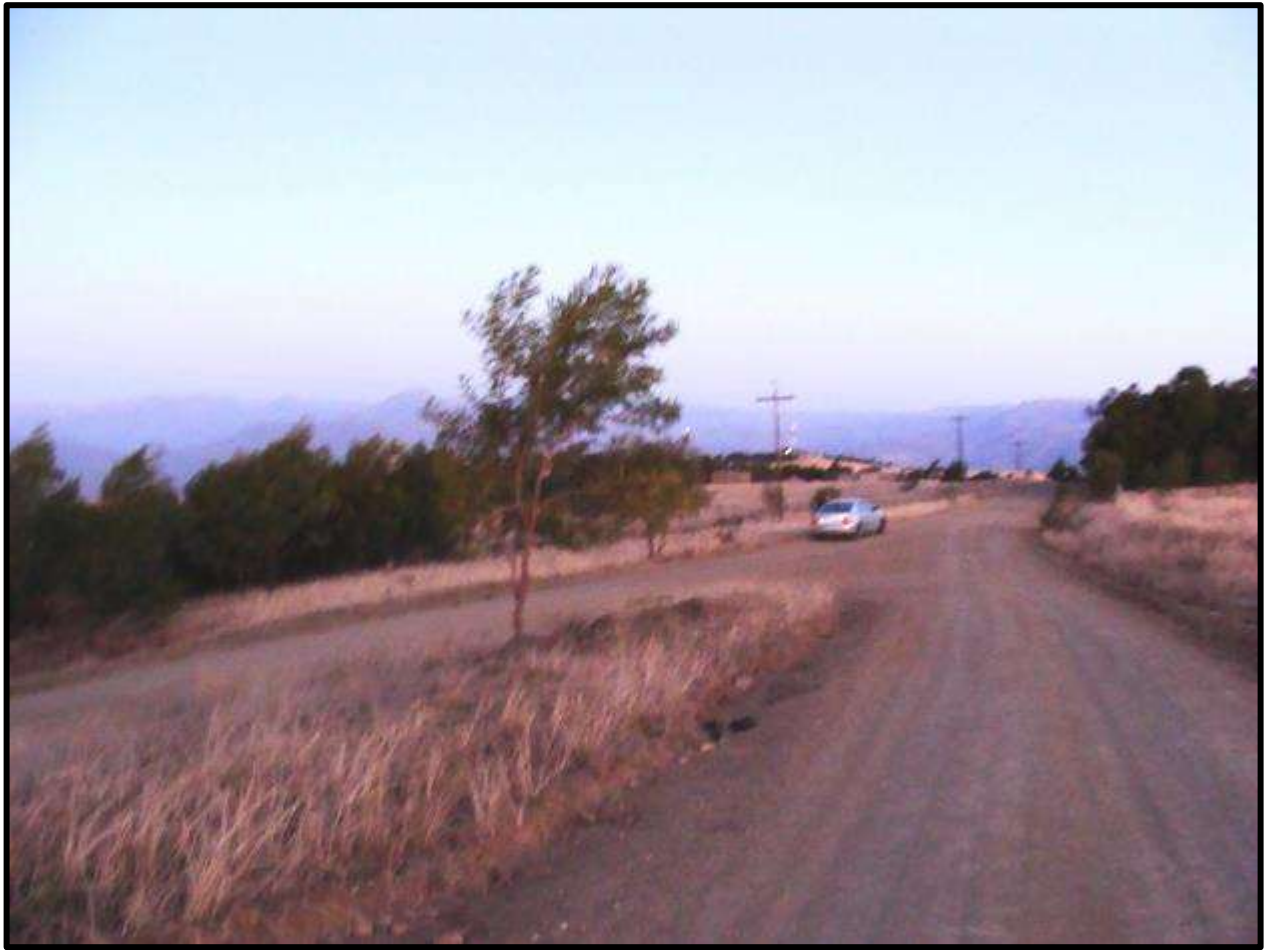
Figure 16: End of the D1269, GPS co-ordinates 28° 42' 55.80" S, 30° 33' 15.58" E
