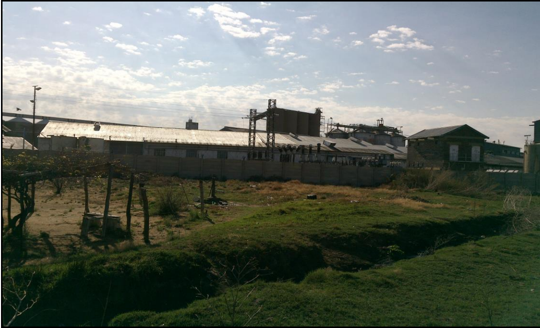
Figure 4: View of Senwesco Substation (GPS S27 12'07.0" E26 54'43.4")
