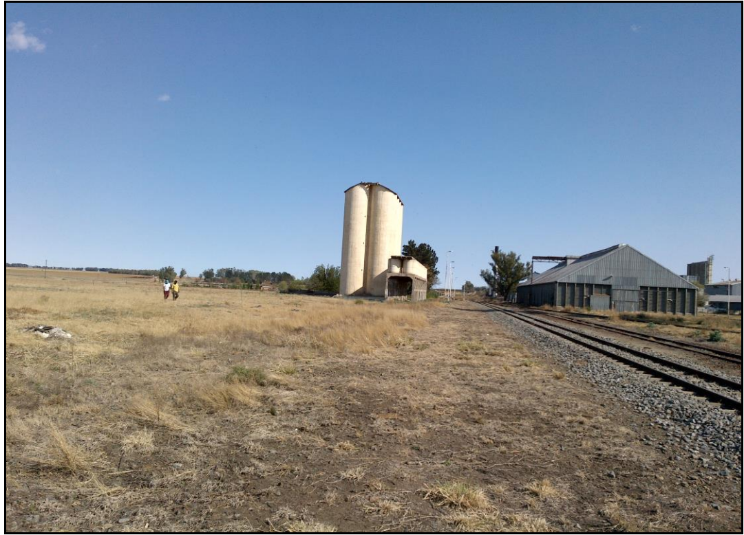
Figure 5: Old Silos on the Southern section of the Senwesco Substation (GPS S27 12'23.3" E26 55'03.1")
