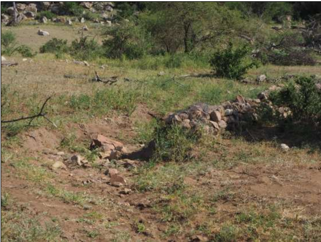
Figure 54. Secondary erosion as a result of the original 2004 anti-erosion measures
