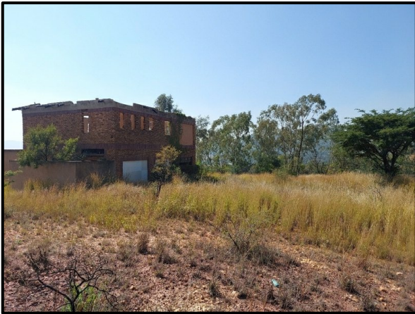
Figure 8.2. General site conditions - Image showing the southern elevation of Hal01.
