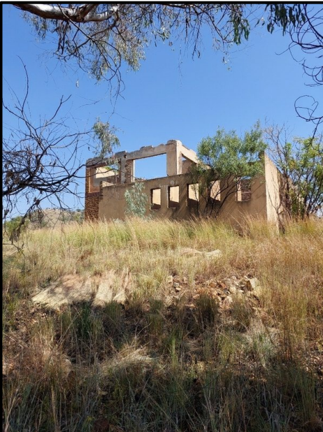
Figure 8.4. Image showing the eastern elevation of Hal01.
