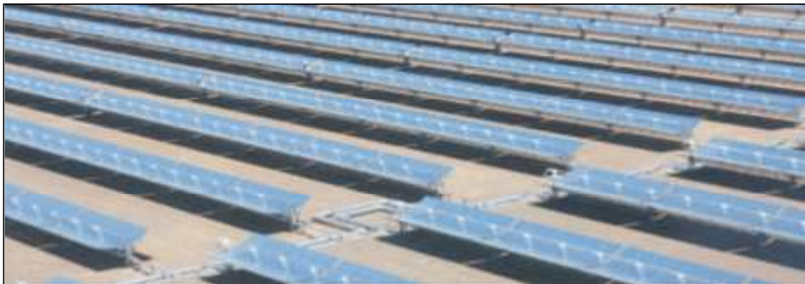
Figure 4. Reflective solar plants (parabolic troughs)
