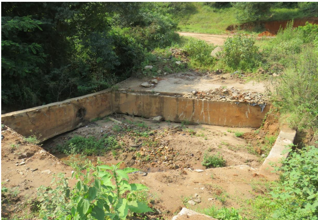
Figure 6: Damaged culvert
