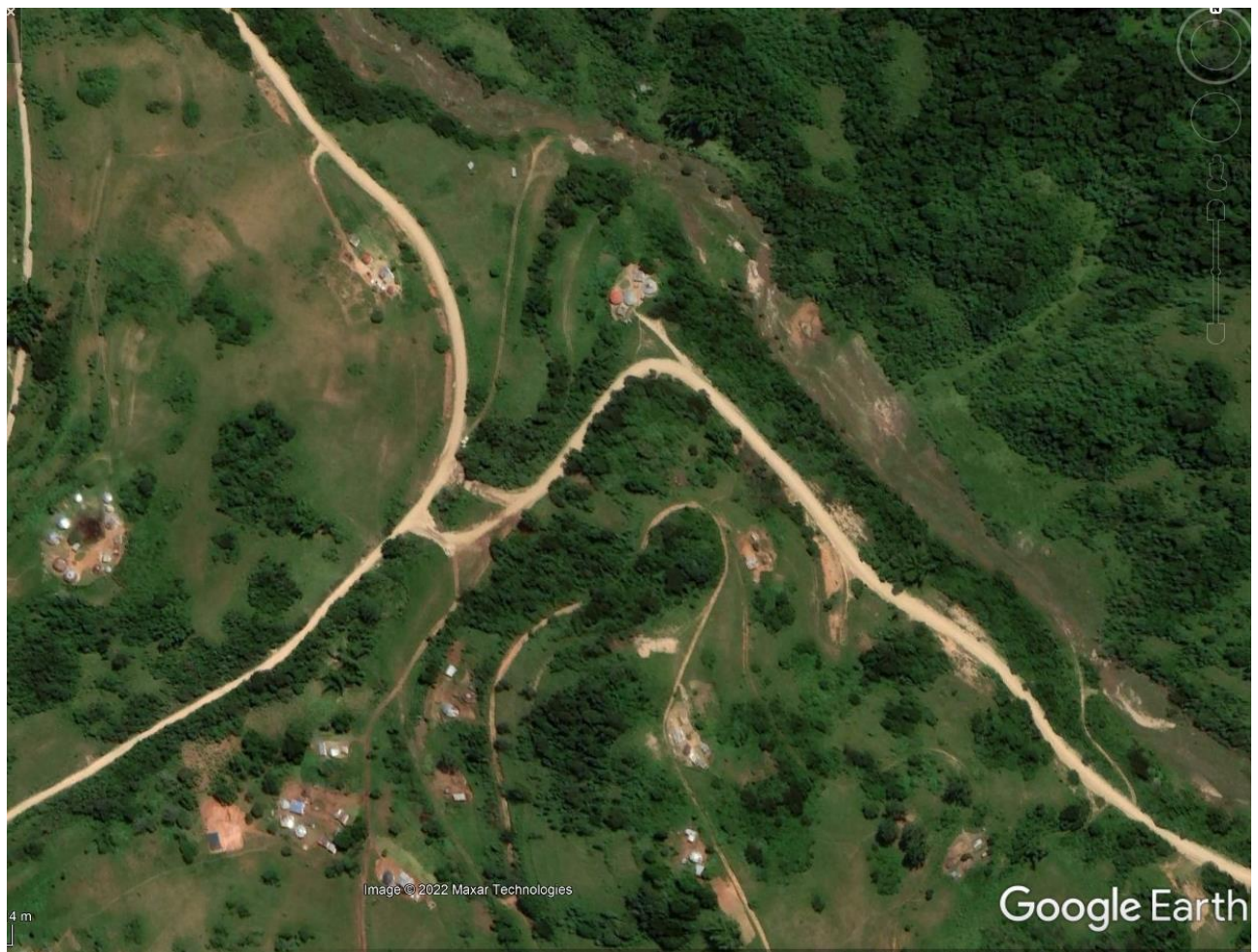
Figure 2: Damaged culvert and earthen structure
