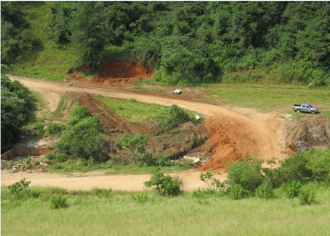
Figure 5: Culvert on left and earthen structure to the right
