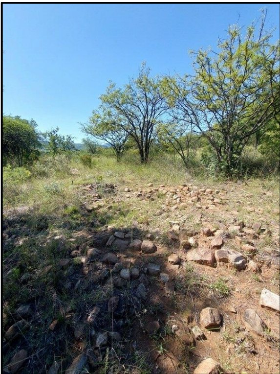
Figure 8.8. Square packed stone foundation or the remnants of a small structure at DD003.
