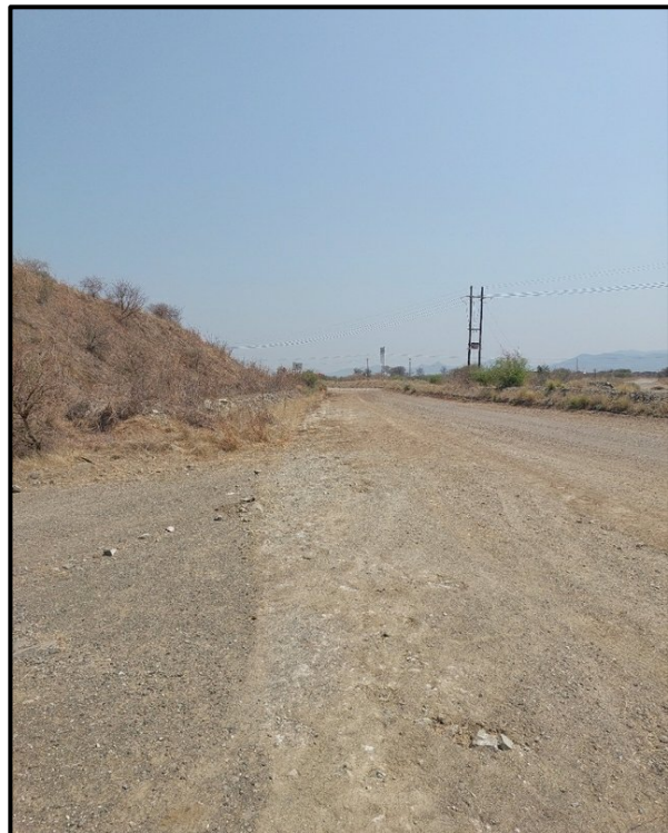
Figure 7.12. Disused existing haul roads running across the project area.
