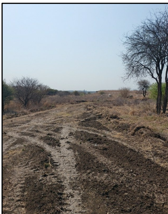
Figure 7.4. Newly made gravel roads run across the project area.
