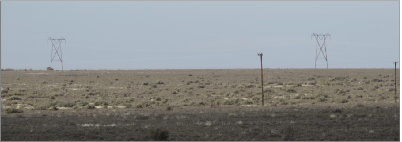
Figure 14: View of existing transmission lines crossing the site.
