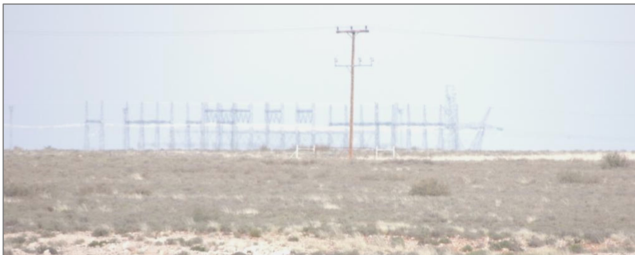
Figure 7: View of existing Cuprum substation
