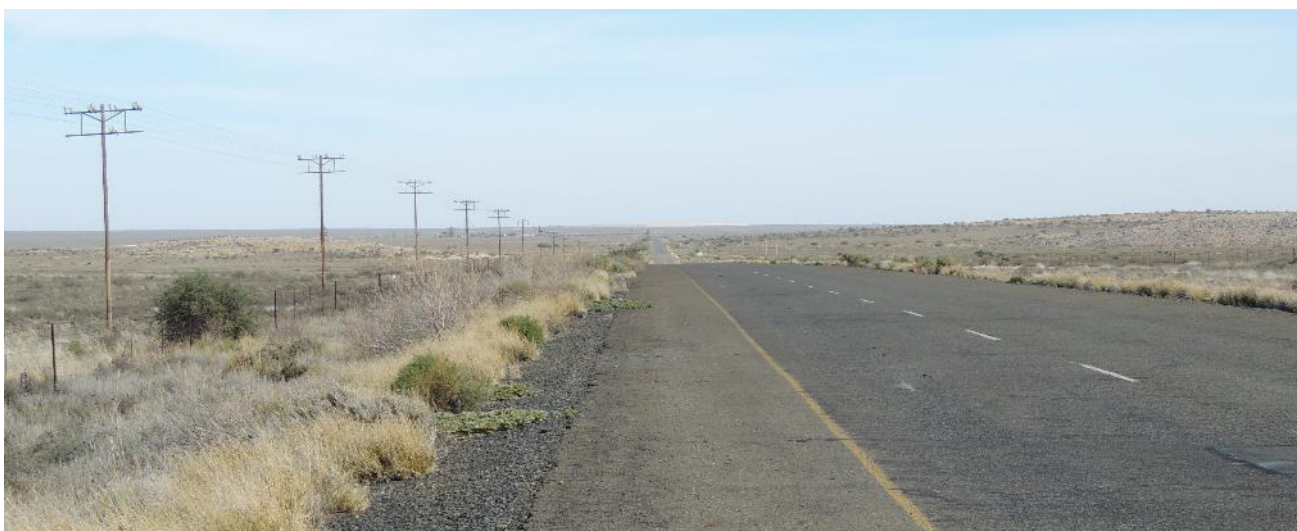
Figure 9: View east of the tarred section of the R357 road
