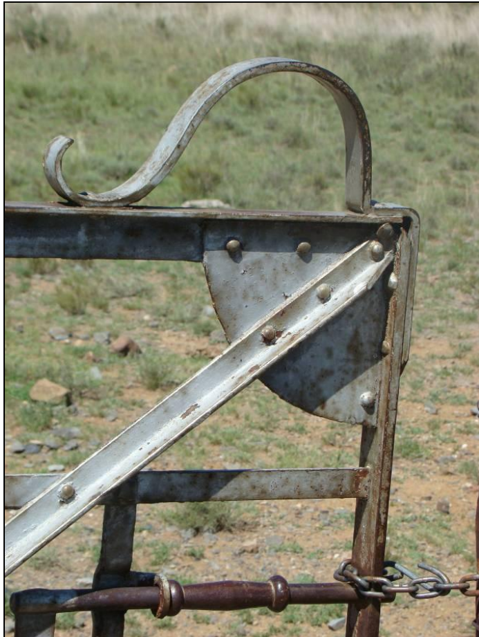
Detail of closing bolt of the fence gate, railway line on Knapdaar 14, Springfontein.
