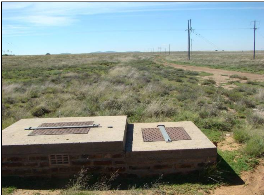
Water pipeline at Knapdaar 14, Springfontein.
