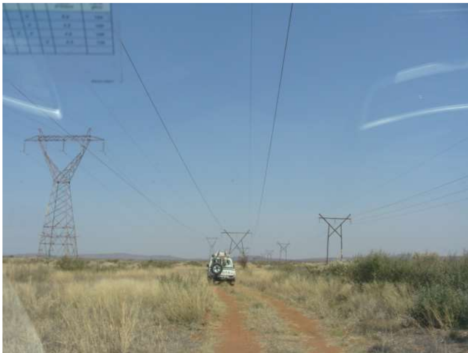
Figure 9: View along the section of the line which will be decommissioned.
