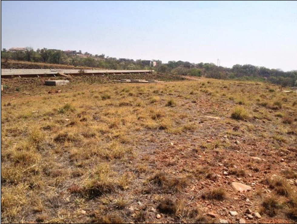
Figure 3-6: Disturbed surroundings at the eastern offset of the rinsing main pipe, the Rand Water reservoir is visible on the left.
