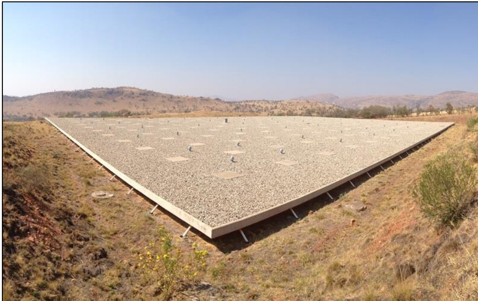
Figure 2-4: View of the existing 100MI Rand Water steel reservoir.
