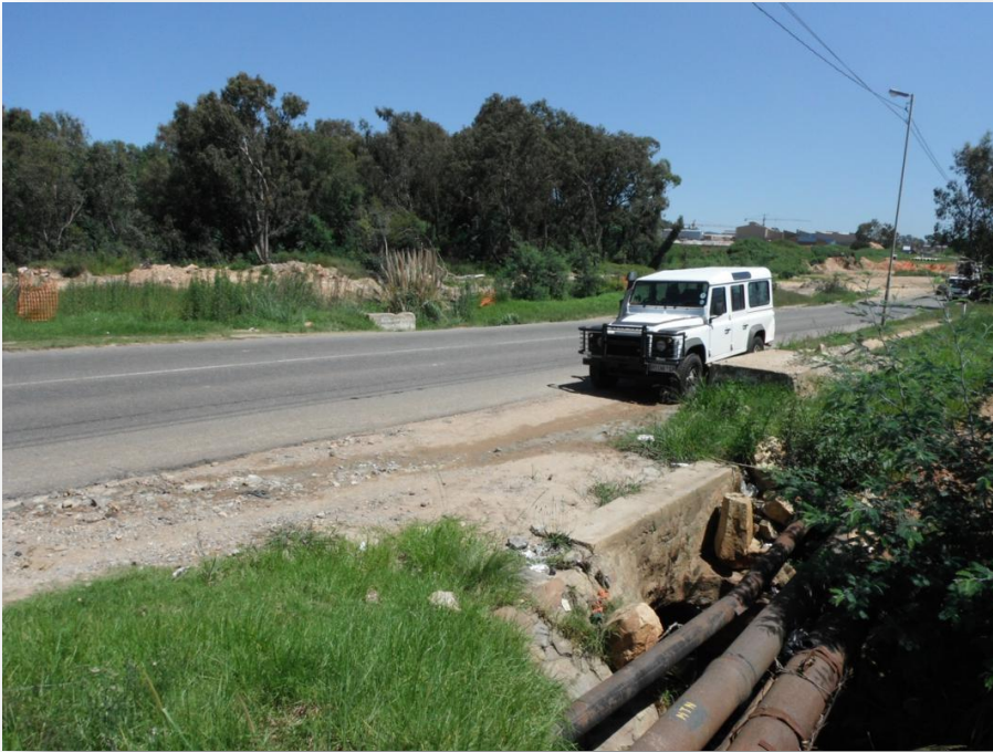
Figure 13 – Culvert and pipe channeling the Elsburg stream under the R29
