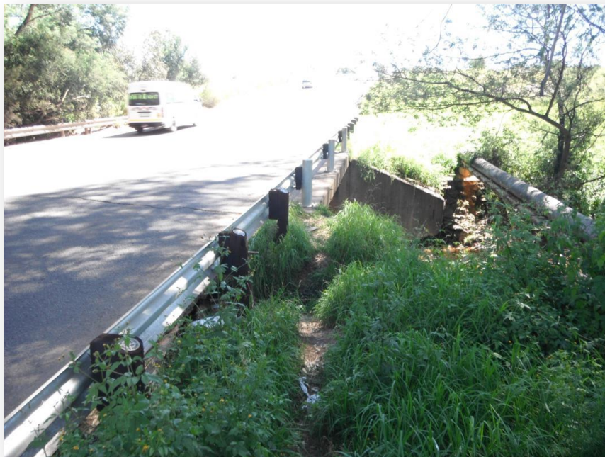
Figure 5 – View of DRD stream bridge on the R29
