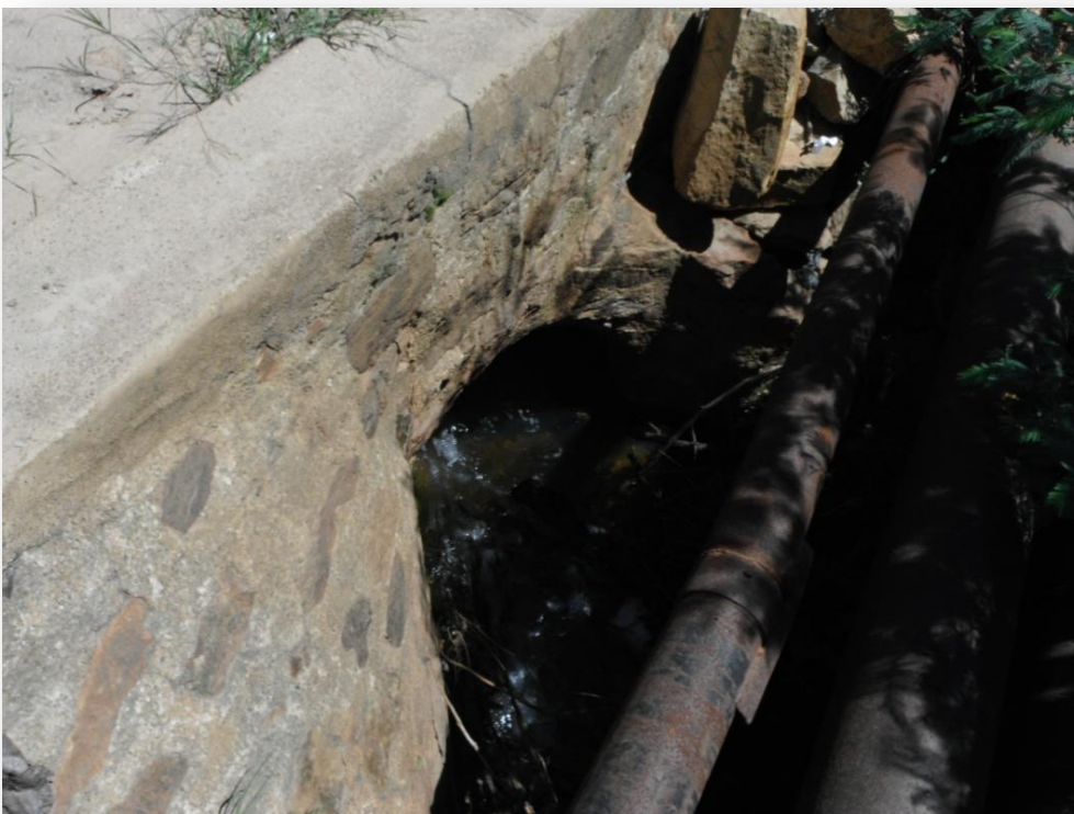
Figure 14 – Close up of stone work on culvert
