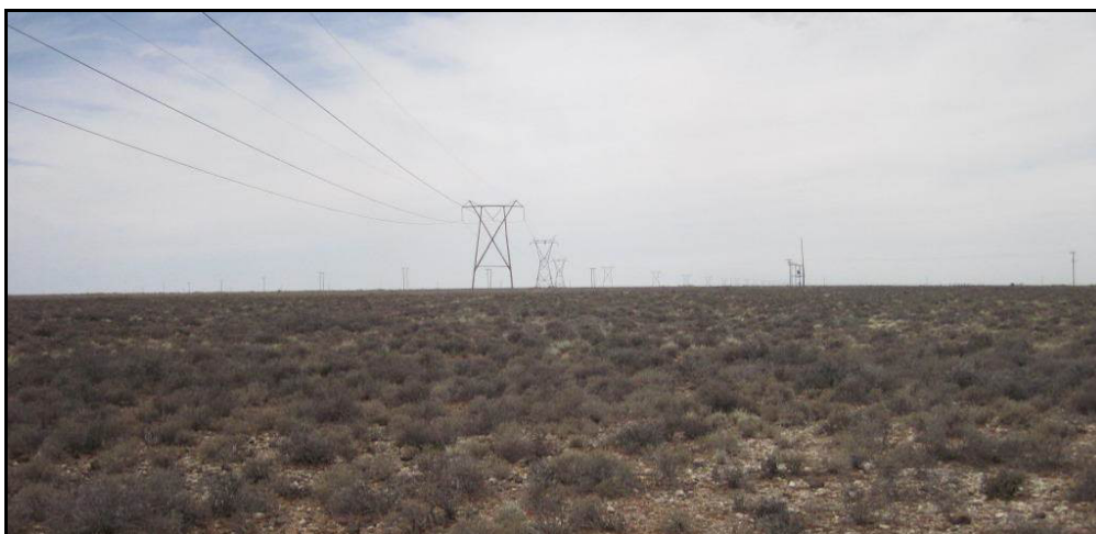
Plate 3: View of the powerlines which cut across the western edge of the property.
