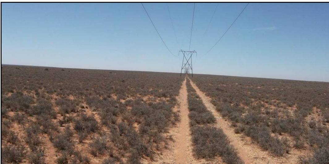
Plate 2: There are two sets of powerlines (and servitudes) which cross the property at right angles.
