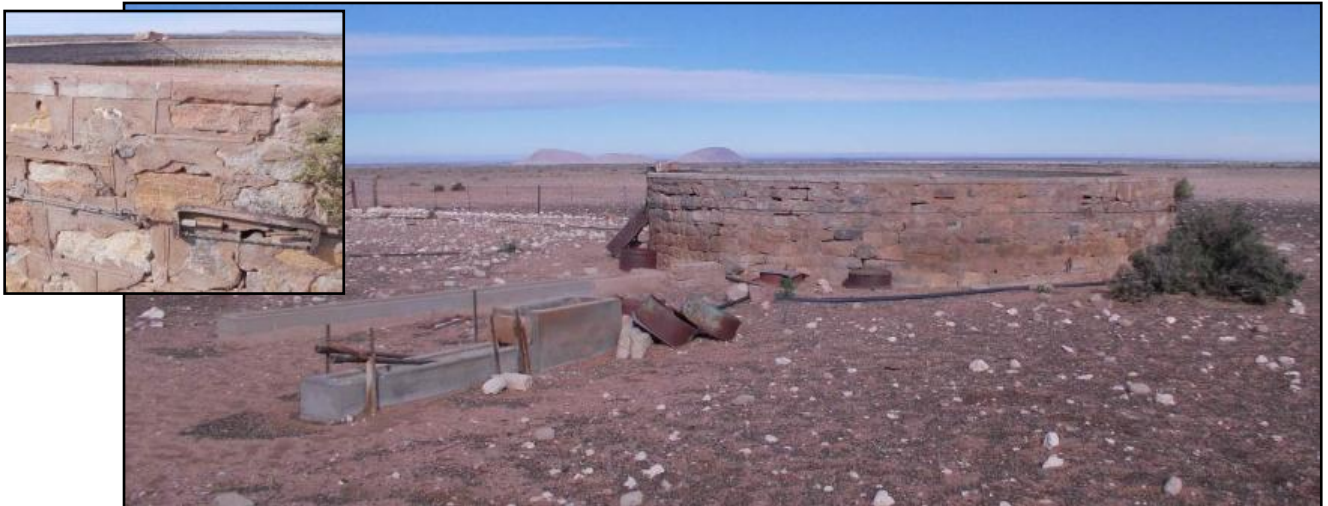
Figure 40: Farm dam at point 016. The inset shows the pointing and a tensioned cable to hold the dam together.
