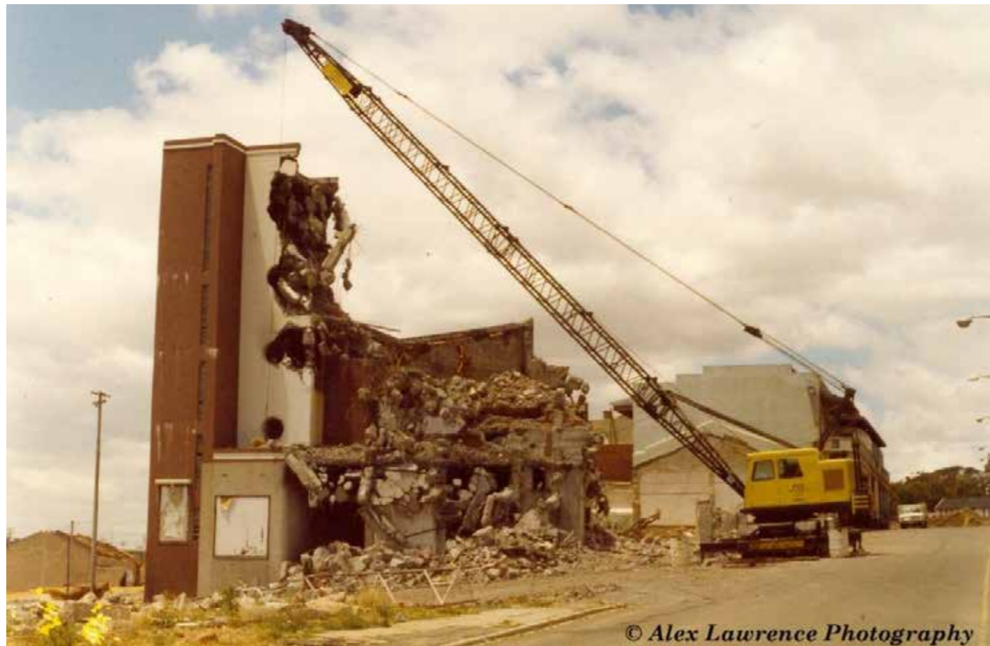
Figure 34. The demolition of the Avalon Cinema (Alex Lawrence in Randle, 2022: 15)
