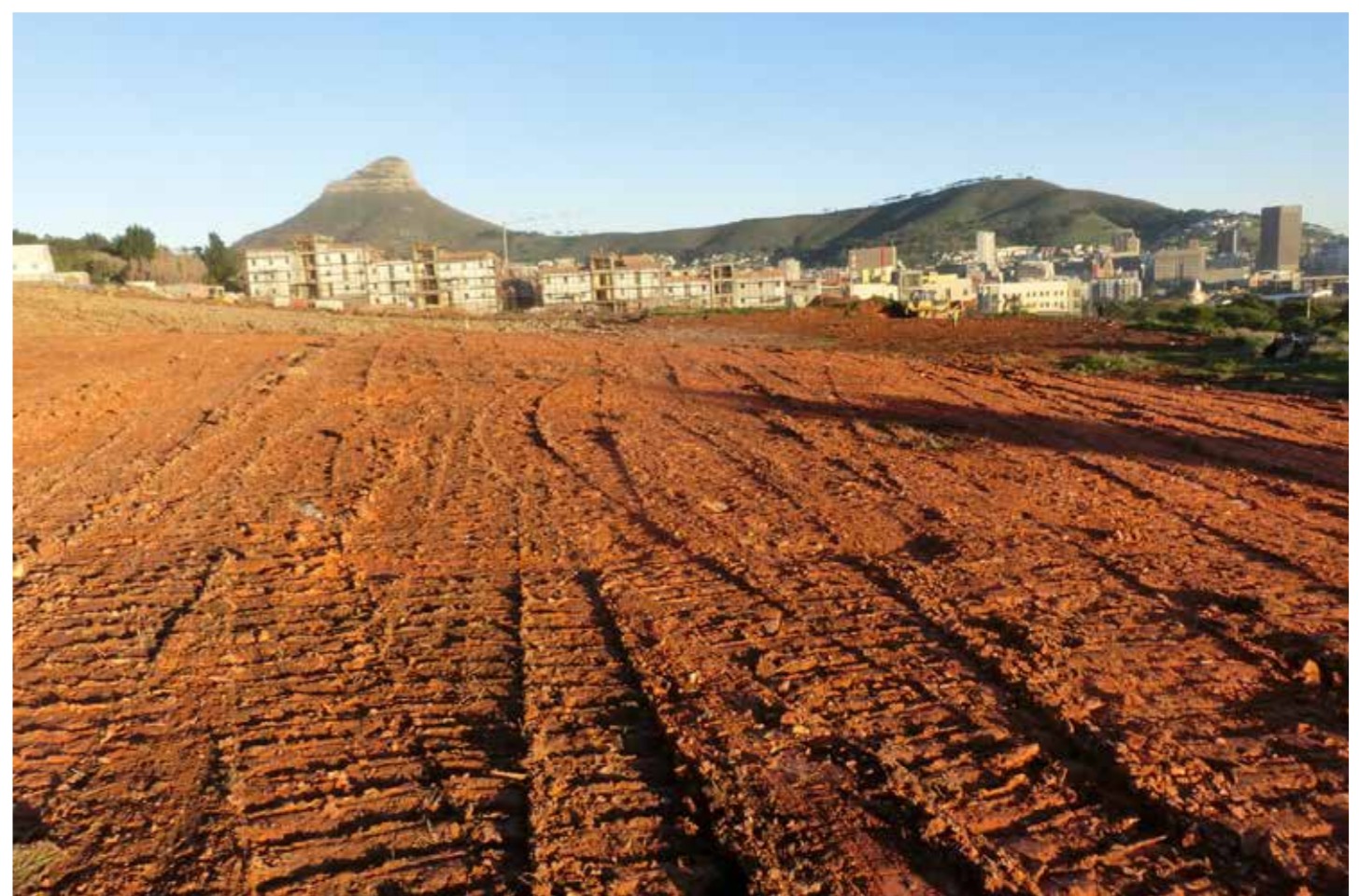
Figure 8. Phase 4 during site levelling, view to west (RSA, 2020)
