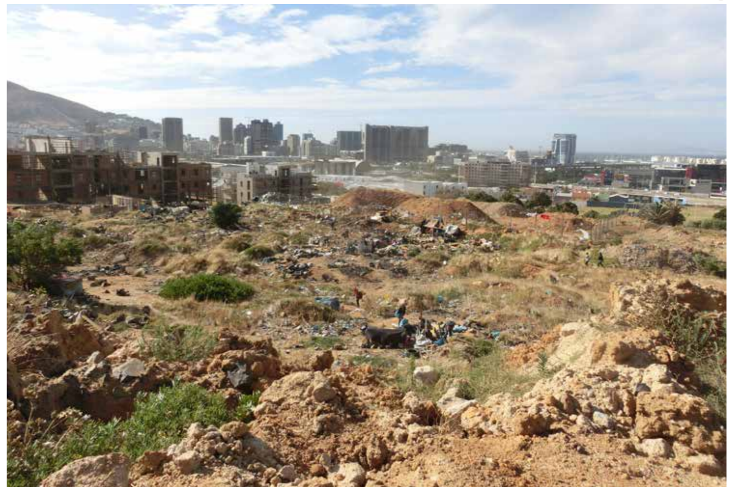
Figure 7. Phase 4 during site levelling, view to north (RSA, 2020)
