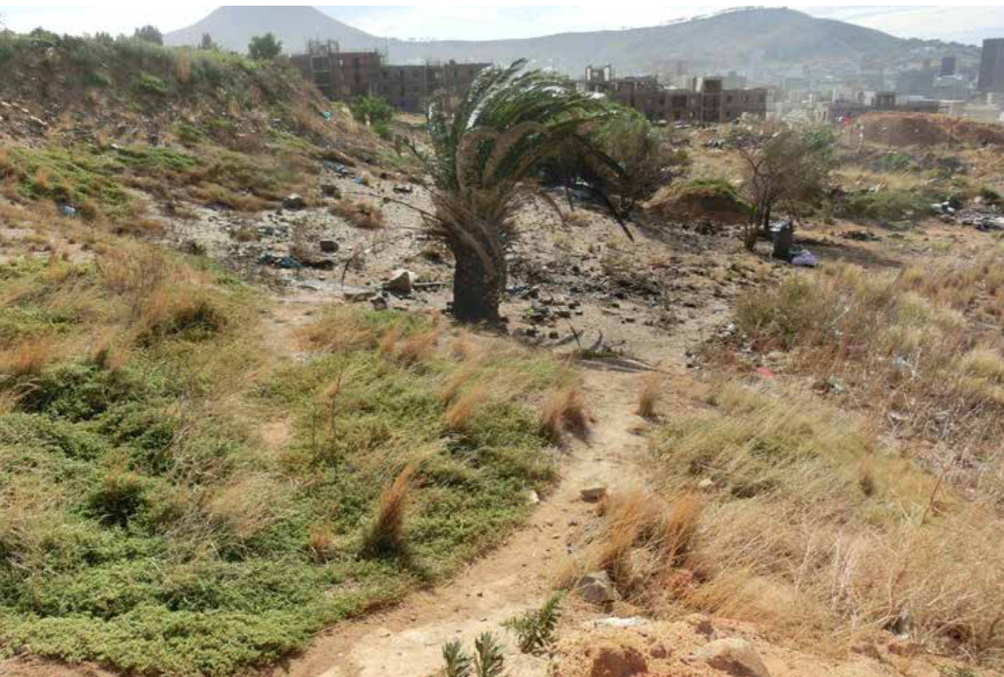
Figure 6. Phase 4 during site levelling, view to west (RSA, 2020)
