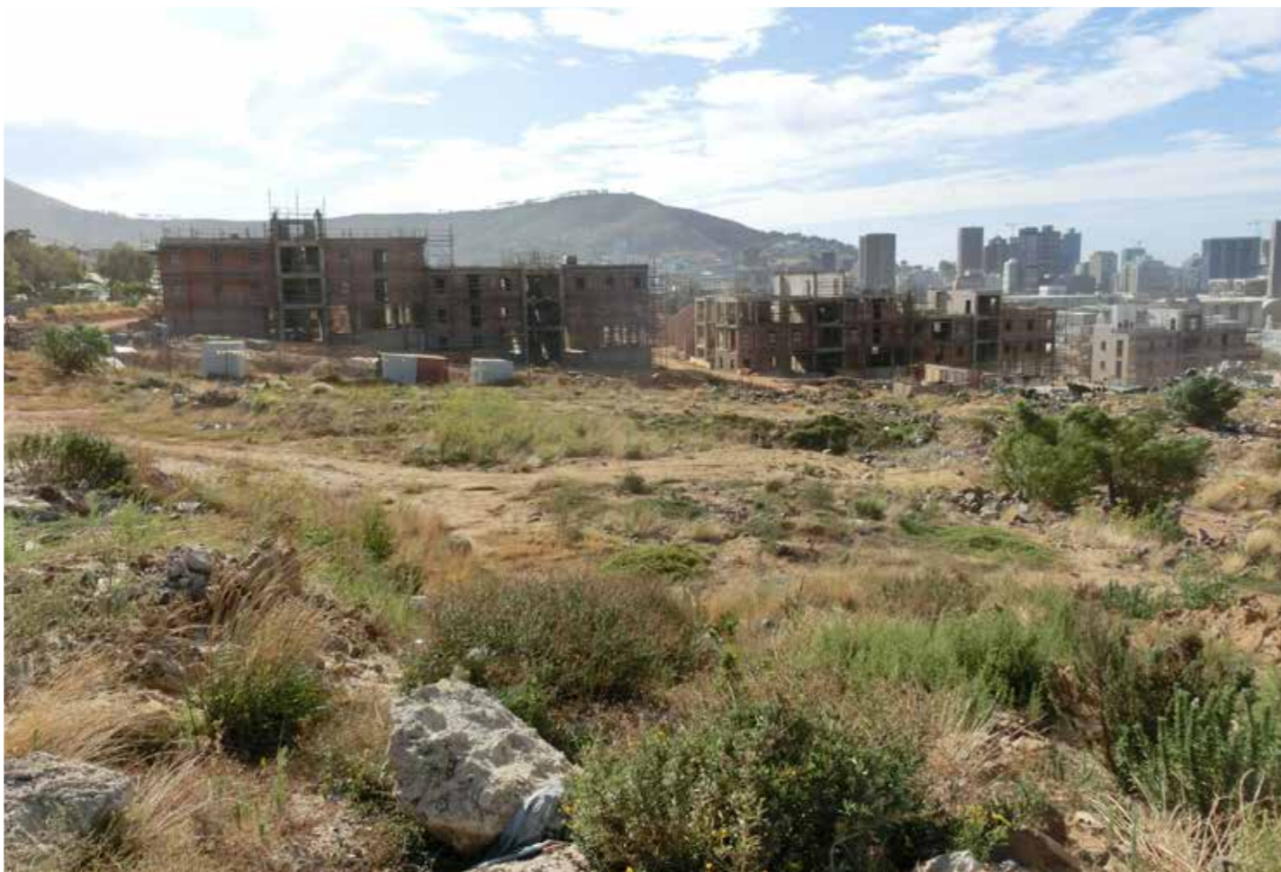
Figure 5. Phase 4 prior to site clearing, view to north west (RSA, 2020).
