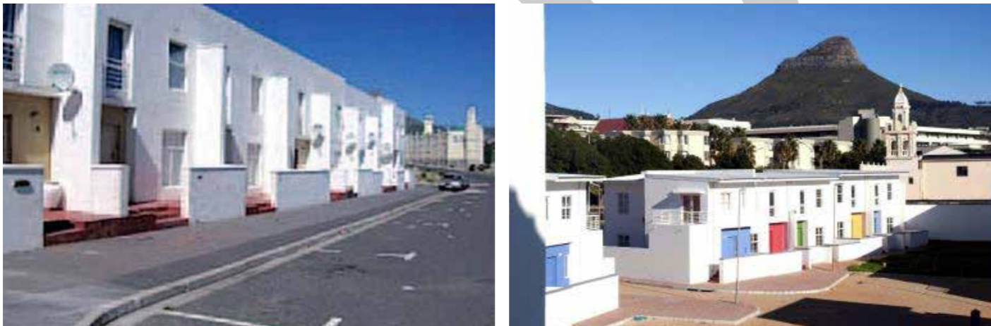
Figure 52. District Six Phase 1 and 2 developments, with row houses offering a choice between duplexes or second floor apartments (iol.co.za, 2011; CoCT, 2021)
