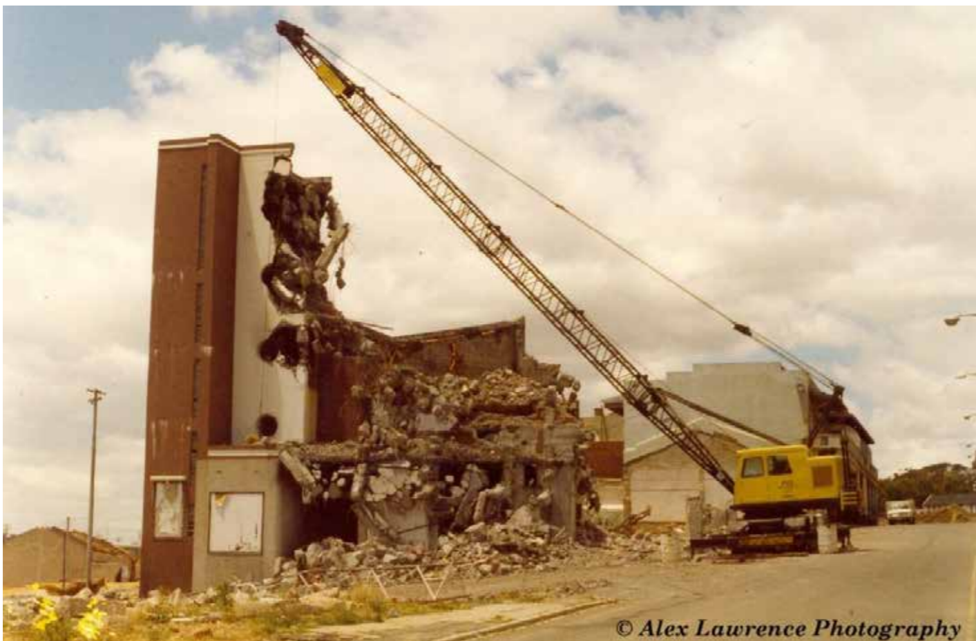
Figure 34. The demolition of the Avalon Cinema (Alex Lawrence in Randle, 2022: 15)
