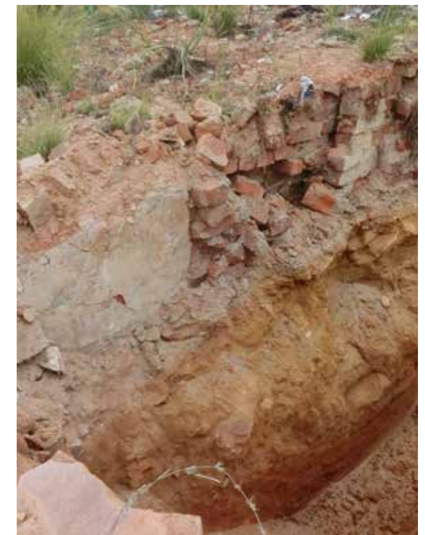
N8 N8 contained disturbed demolition rubble to a depth of 1m overlaying natural deposits.
