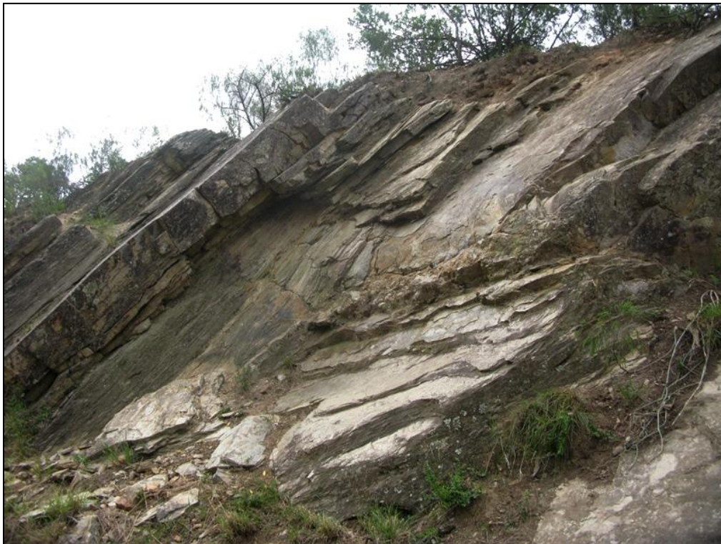
Figure 10. R102 road cutting through folded quartzitic wackes and phyllitic pelites of the Sardinia Bay Formation, c. 1 km west of Van Stadensrivier (Loc. 025).
