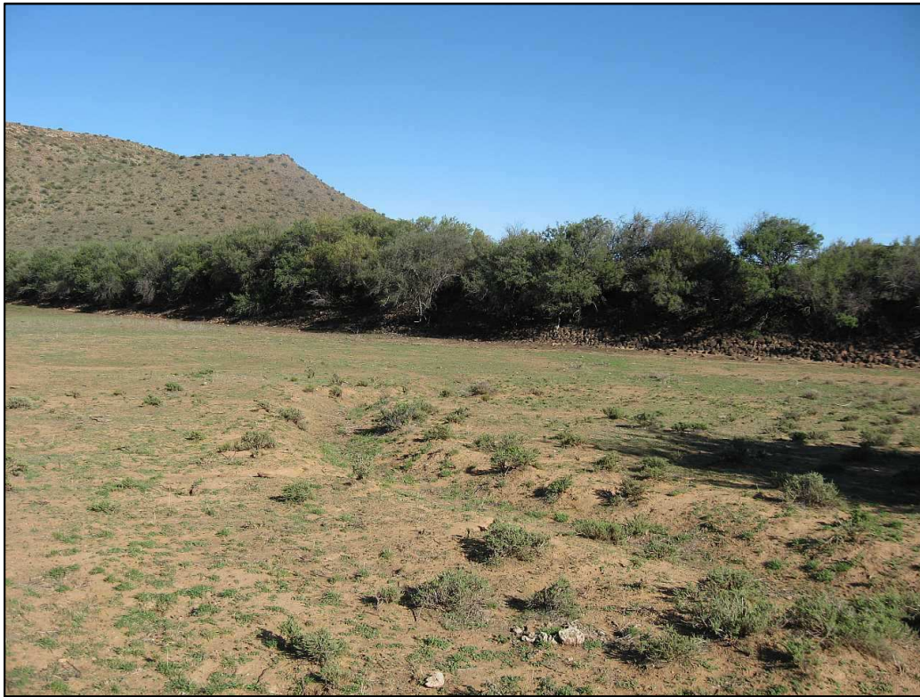
Figure 16 – View of dam wall
