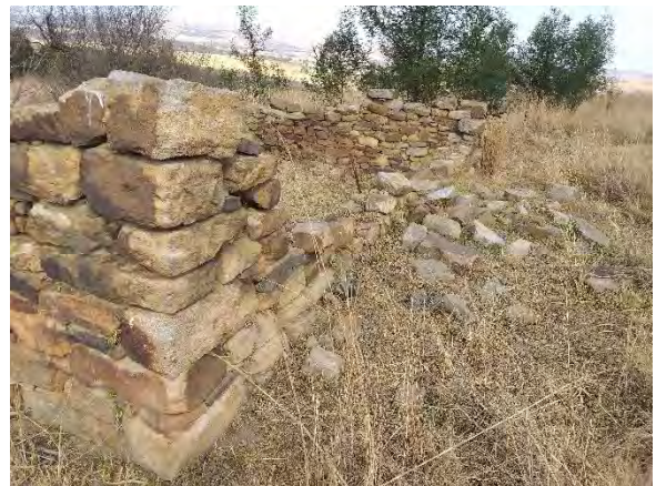
Remains of one of the farm labourers houses at HST-002
