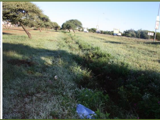
Plate 2: Water drainage Canal.
