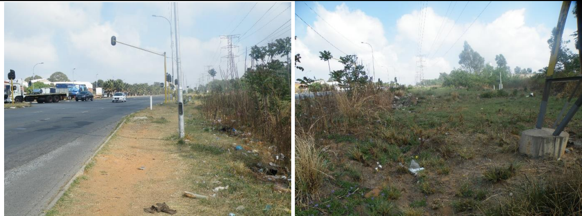
Figure 8: Most northern extent of the pipeline route where it crosses over Main Reef Road into degraded vegetation
