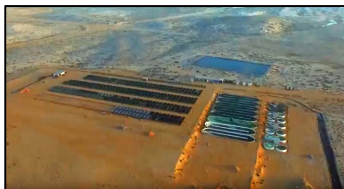
Figure 3. The existing abalone farm and solar dam, showing yellow made ground.
