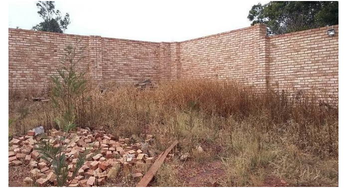
North eastern boundary wall of subject area
