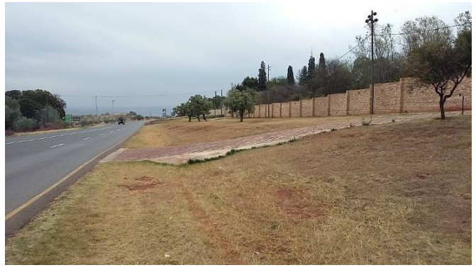
Access to site of R563 (Hekpoort / Krugersdorp Road)
