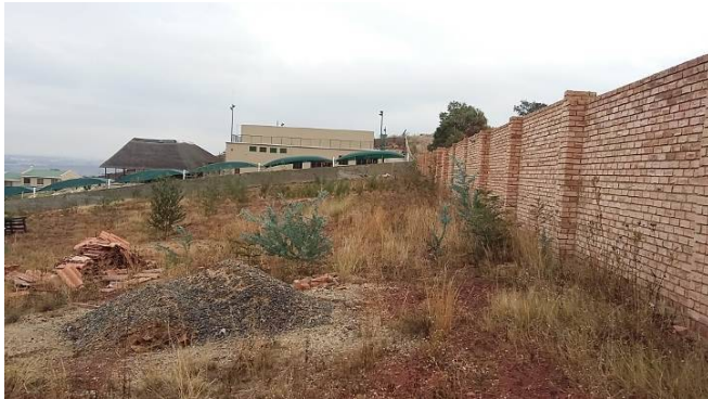
Northern boundary wall of subject area
