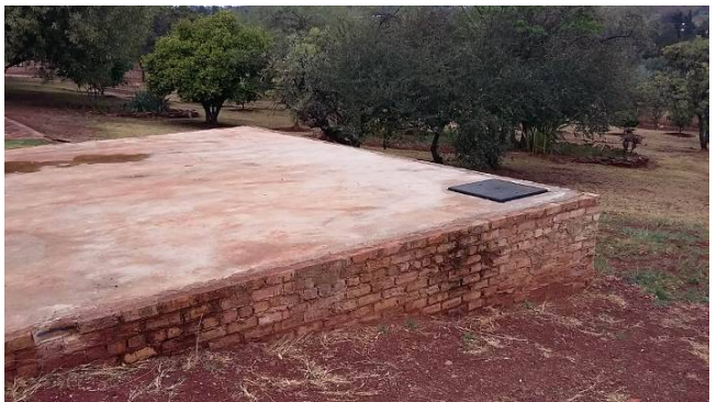
Existing conservancy tank
