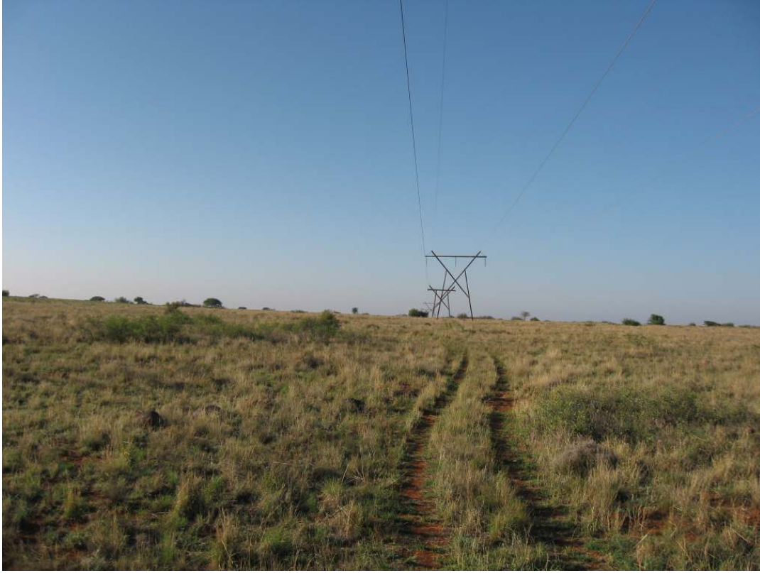
Photo 3: View of the “Jacobsdal/Kimberley” 132kV power line which crossed the site.
