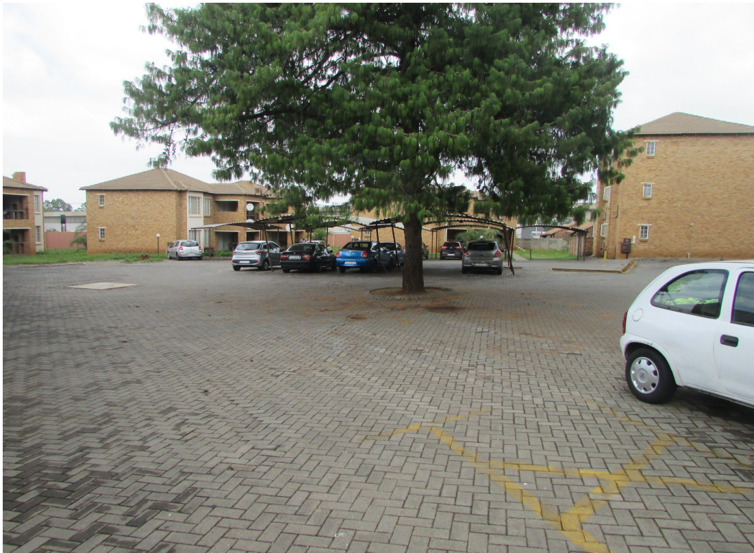
Figure 7: Another part showing parking lots and units.
