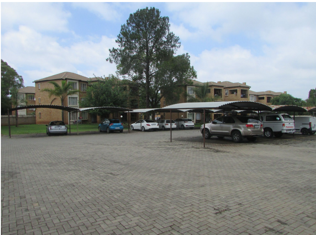
Figure 5: View of parking area and more of the existing units.
