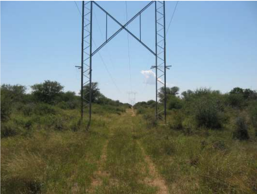
Photo 2: View of the power line across the property.
