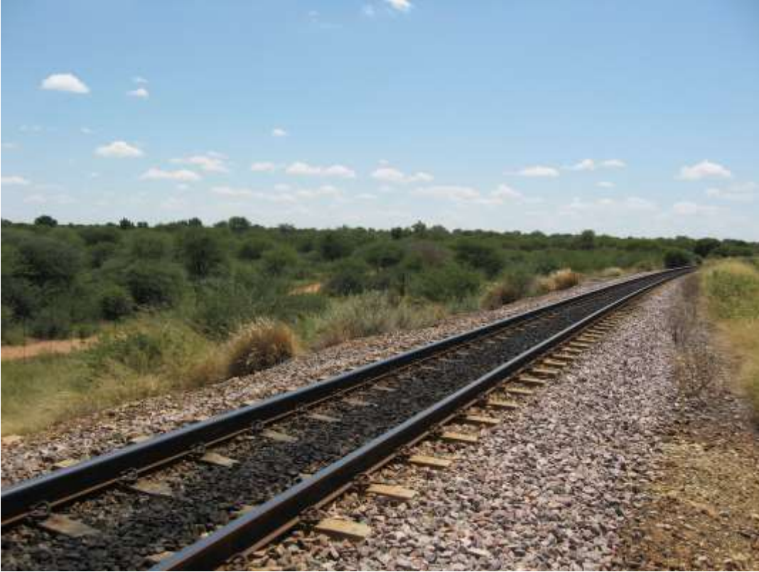
Photo 1: View of the railway line on the southern side of the property.
