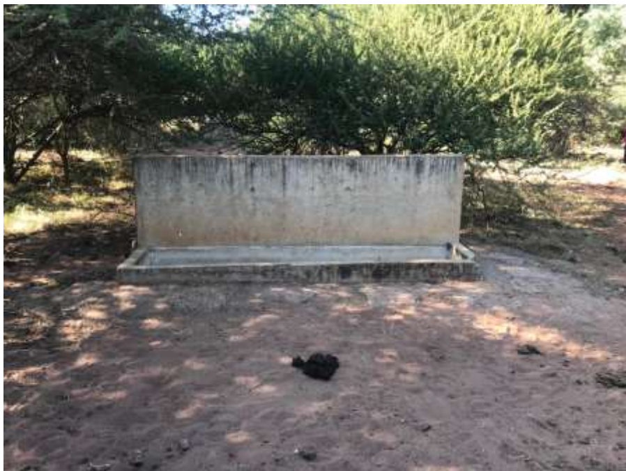
Figure 6: Old Cattle Water Drinking Trough on site.
