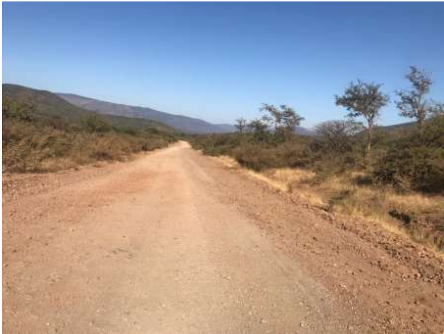
Figure 4: View of the access road
