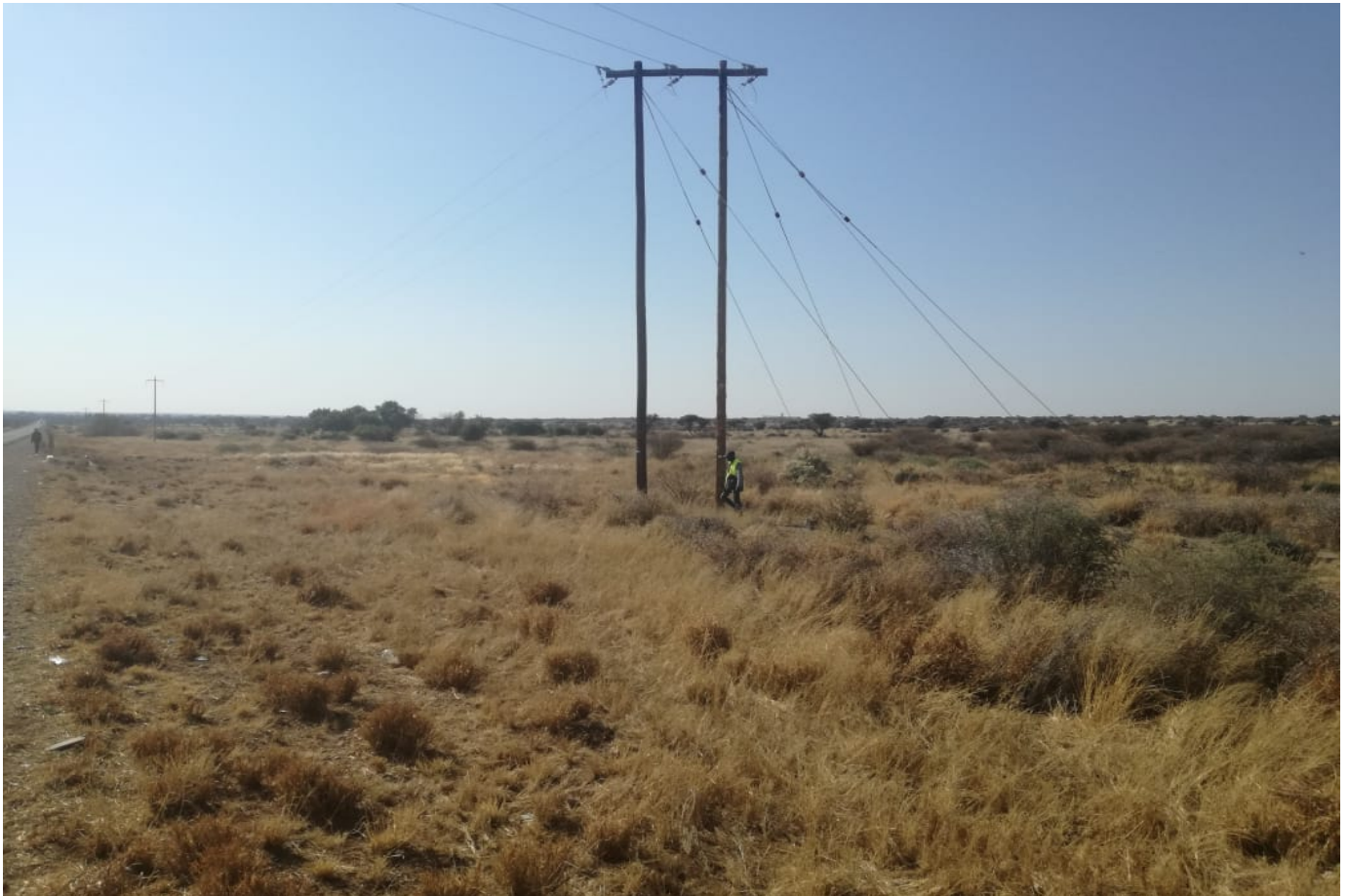
Figure 1: View of pole where the powerline will T-off.
