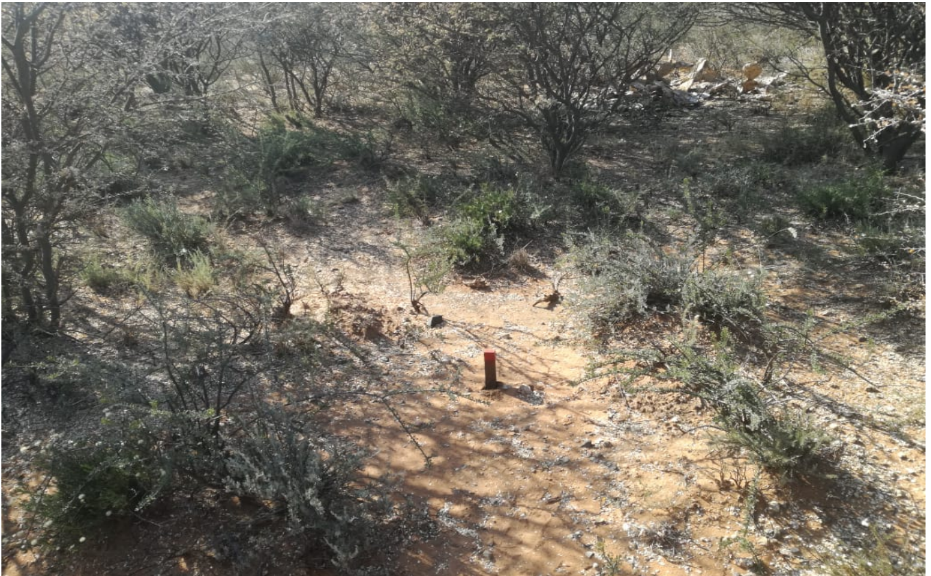
Figure 4: View of powerline pole position marked by a red peg.
