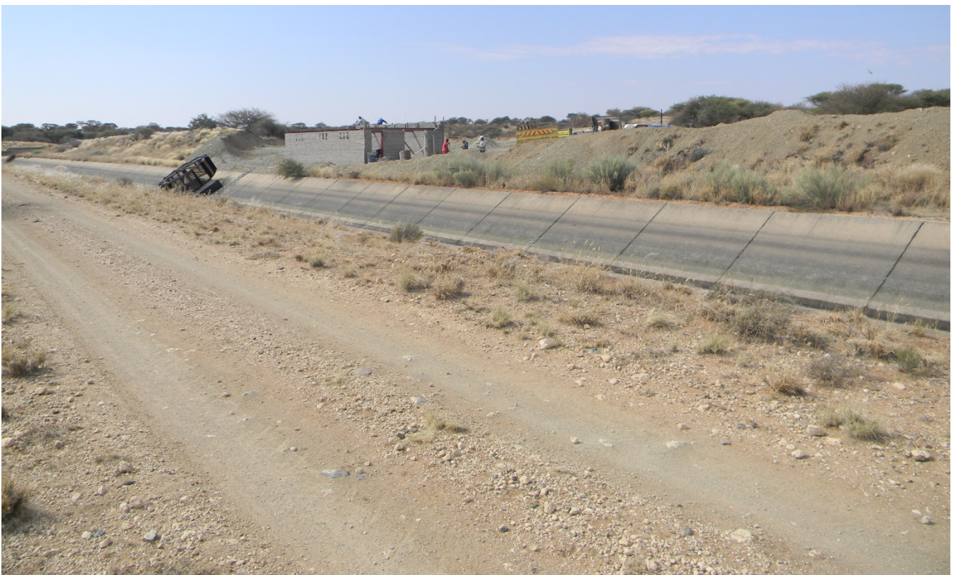
Figure 7: View of terminal position at new pump house across the canal
