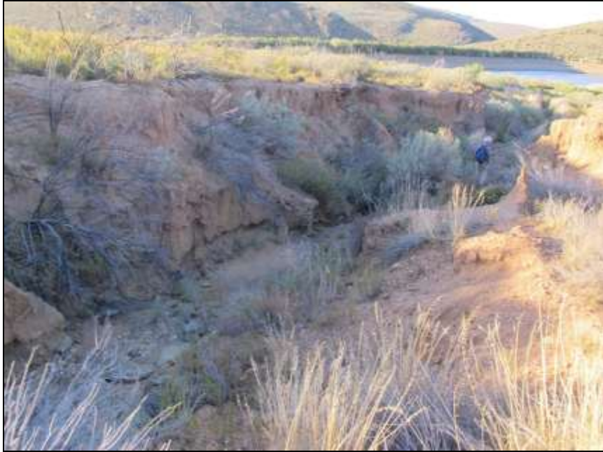
Figure 5: View northwards along the donga to the west of the affected area of pit 25. Slabs of weathered Bokkeveld shale are visible in the bottom of the donga.
