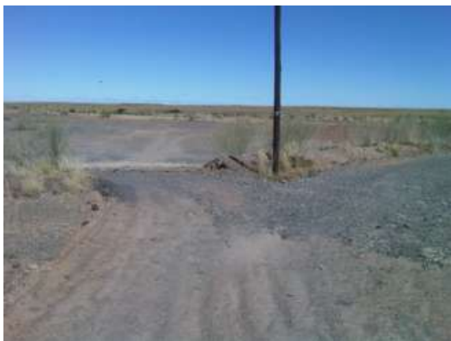
Looking southeast towards the existing borrow pit showing the access road (left), farm road (right) and electricity pole (April 2011). Operations is to reinforce ground around the pole and excavate mine from where it will not pose a risk to the electricity line.
