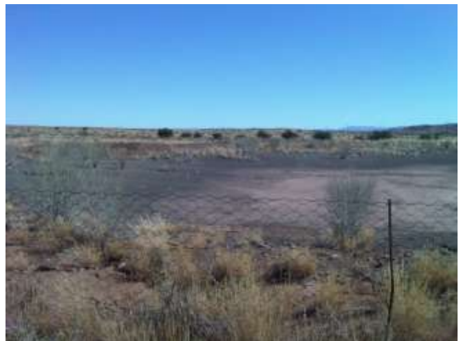
Looking west at the basin of the existing dam which will be deepened as part of the proposed activities (April 2011).
