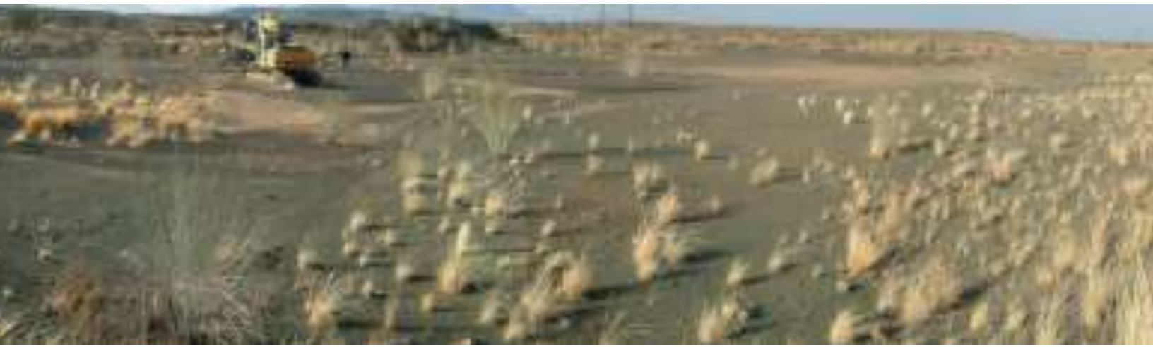
DR 02308/12.9 View from existing dam embankment towards borrow pit extension area
