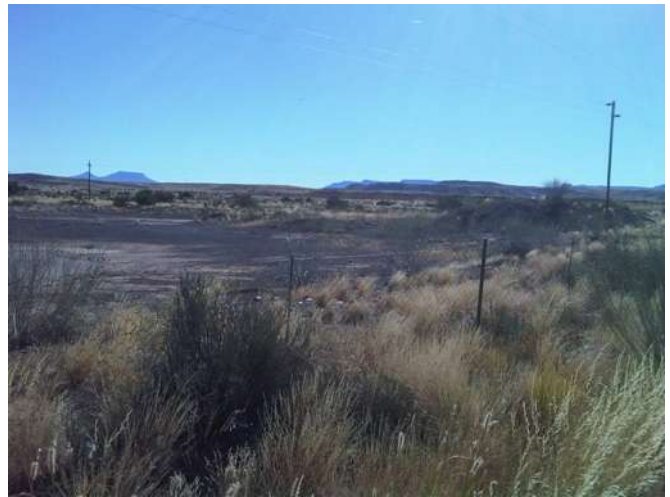
Looking northwest across the site of the existing dam which will be expanded under the proposed programme (April 2011).
