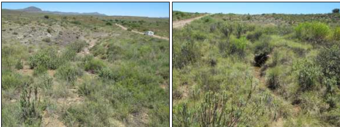
Figures 3 and 4: Pit 30 – view of the eastern side of the study area showing the existing quarry with exposed Beaufort Group siltstone (view towards the south) and disturbance caused by water erosion (view towards the north). The existing quarry lies towards the top of the slope in the photo to the right.
