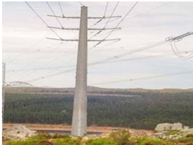
Figure 9: An Example of Powerline Picture (Monopole Structure)
