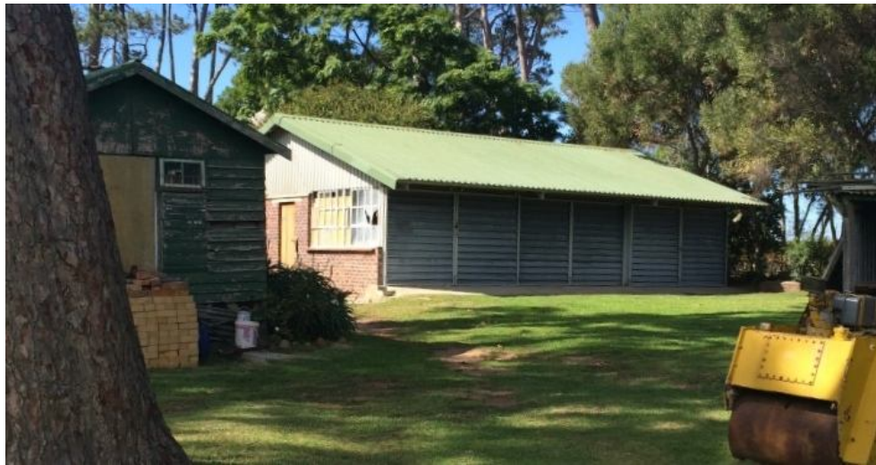
Figure 20: Shed and workshop
