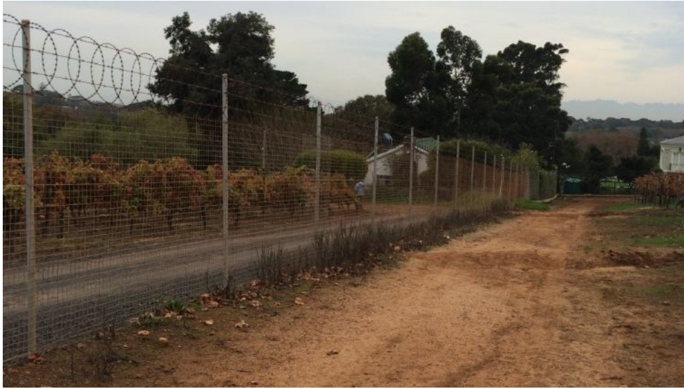
Figure 33: Un-screened section of the fence
