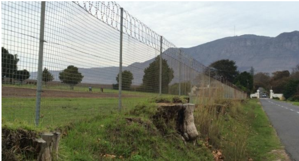
Figure 25: A tall weld-mesh security fence topped with razor wire runs along the section of the road from the main entrance to the dwelling in the western corner where it meets the painted and plastered masonry wall
